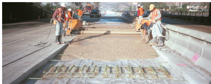
Full-depth overnight replacement of highway pavement
