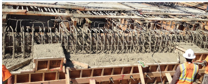
Bridge hinge reconstruction in San Francisco
