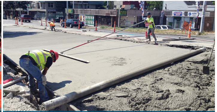
(b) Placement and finishing
