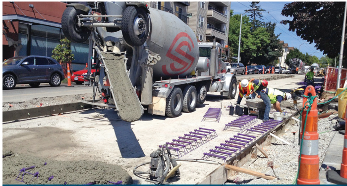
(a) Concrete placement using ready mix truck
