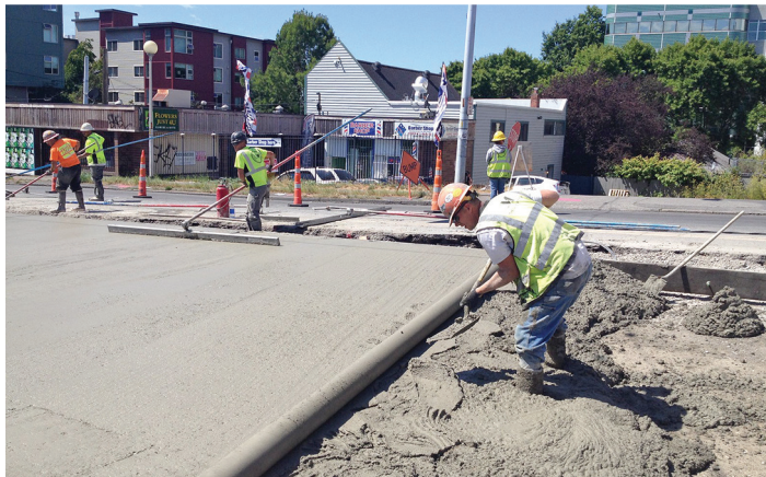
(c) Placement and finishing
