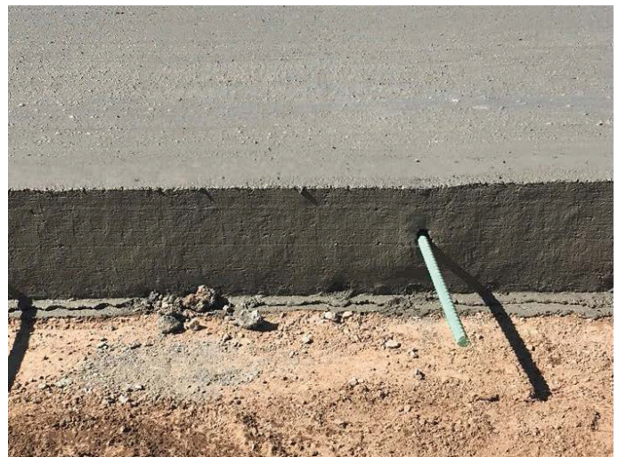
Figure 5. Finished edge with inserted tie bars
