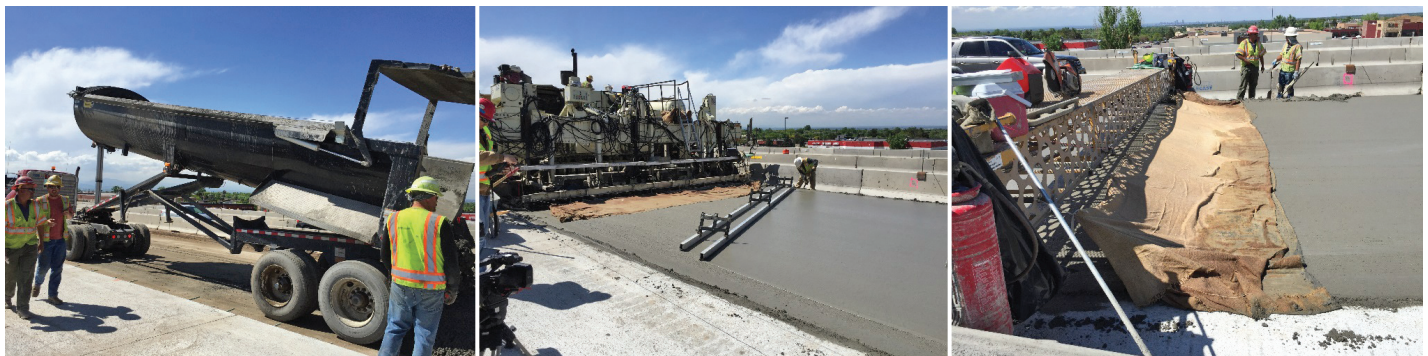
Figure 4. Concrete placement, finishing, and texturing of C-470
