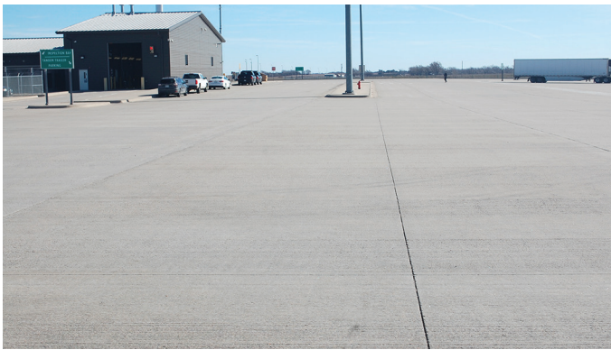
Figure 15. Finished pavement showing joint condition (2024)
