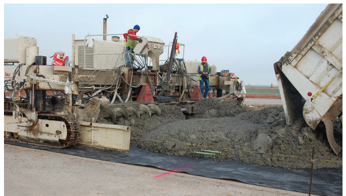
Figure 9. Slipform paving – front of paver
