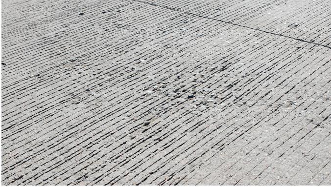
Figure 14. Surface texture inconsistency
