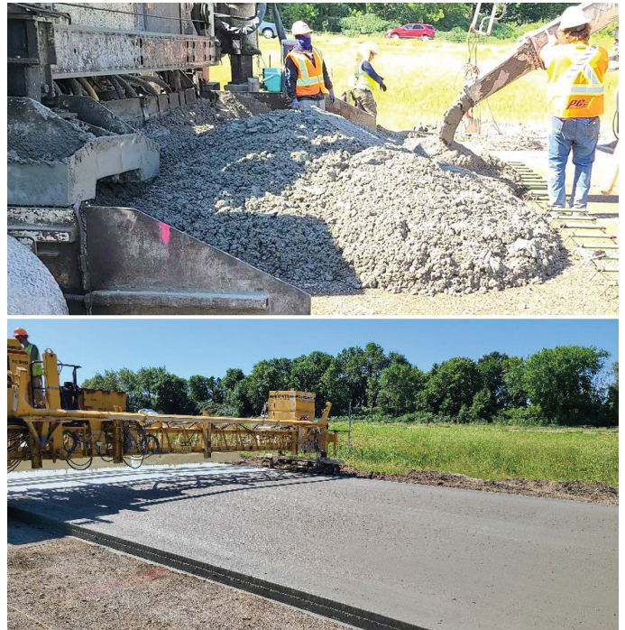
Figure 4. Cell 2219 during construction, with the mixture in front of the paver (top) and the surface texture after placement (bottom)
