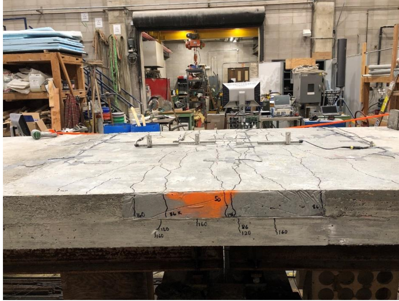
Figure 24. Crack patterns in the depth of the link slab at the ultimate stage
