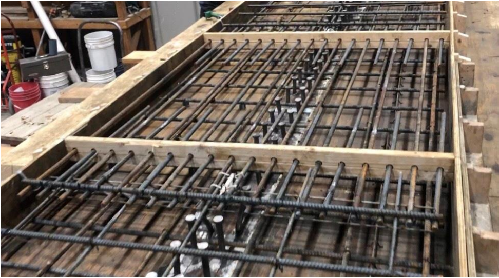
Figure 15. Reinforcement in the link slab
