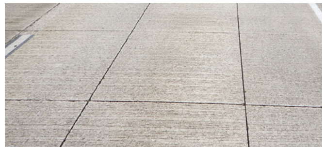
Figure 50. Typical joint condition on US-425 near Ferriday, Louisiana (2019)
