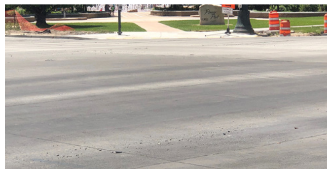
Mitzi McIntyre, CTS Cement, used with permission
