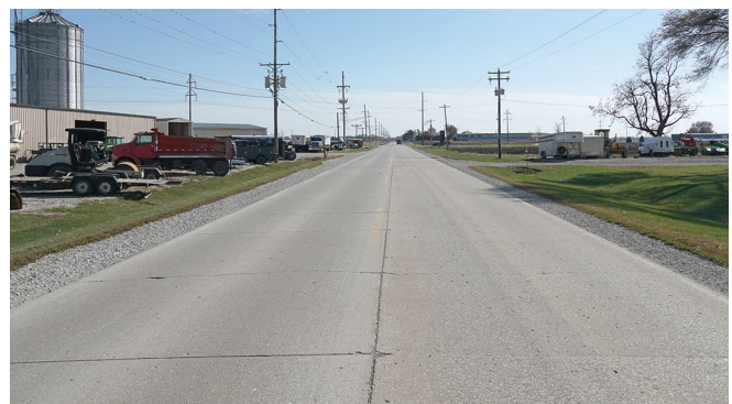
Figure 17. CR-56 near Peru, Illinois, after 48 years (2020)
