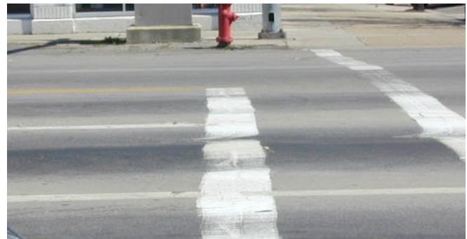
Mitzi McIntyre, CTS Cement, used with permission
