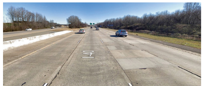
Figure 59. Full-depth patches on eastbound I-40
