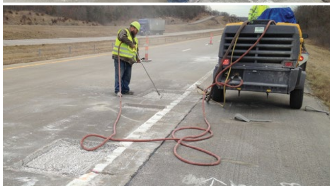
Figure 5.17. Media blasting (top) and air blasting (bottom) of PDR area
