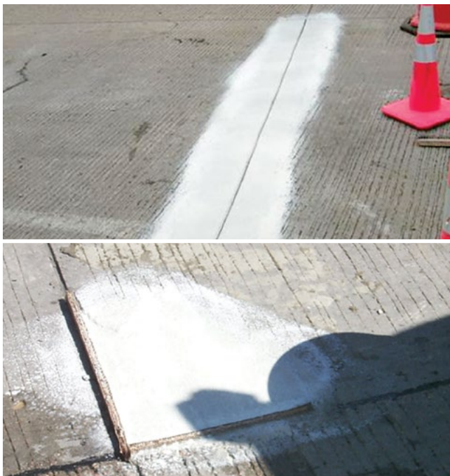
Figure 5.27. Completed PDRs
