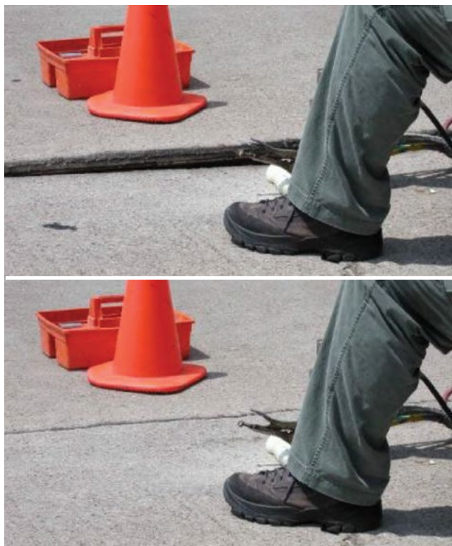
Figure 4.12. Settled slab before (top) and after (bottom) slab jacking
