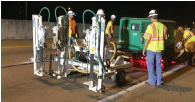
Figure 4.17. Drilling holes for polyurethane foam installation on I-24 West in Tennessee
