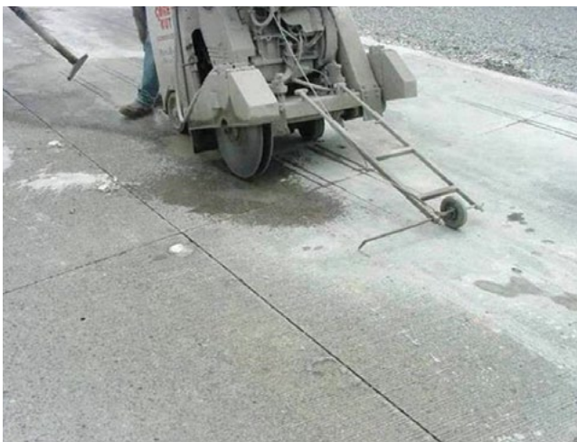
Figure 8.9. Equipment to cut a single dowel bar slot
