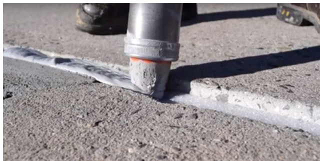
Figure 10.16. Close-up of silicone sealant installation
