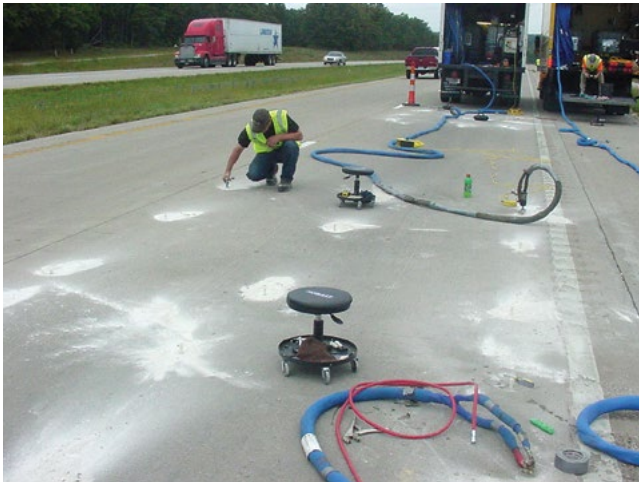
Figure 4.5. Polyurethane stabilization hole pattern
