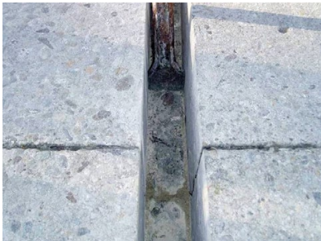
Figure 8.13. Leveling the bottom of the dowel bar slot
