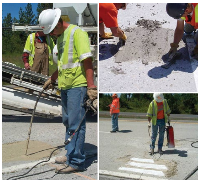
Figure 8.21. Patching material placement: consolidation (left), finishing (top right), and curing compound application (bottom right)
