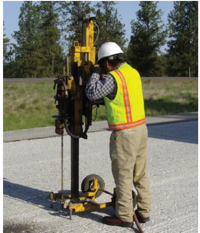
Figure 4.6. Drilling polyurethane injection holes
