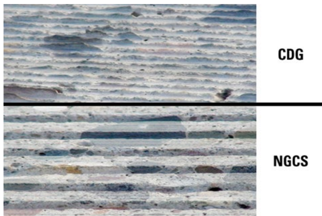
Figure 9.18. Comparison of surface textures produced by CDG (top) and NGCS (bottom)
