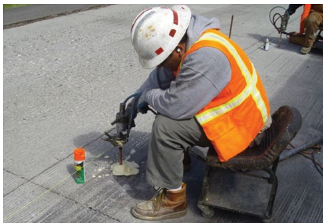
Figure 4.7. Injecting polyurethane for slab stabilization
