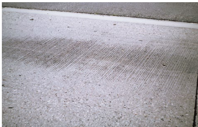
Figure 9.10. Holiday on a diamond-ground surface
