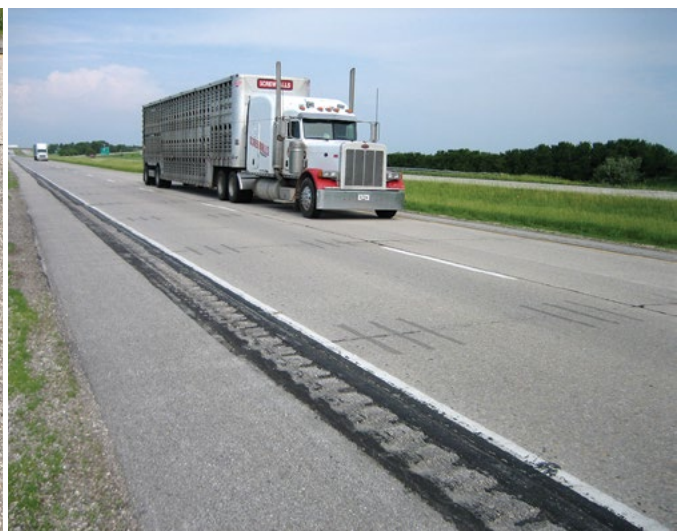
Figure 9.4. Previously overlaid concrete pavement on US 20 in Iowa restored via patching, DBR, and diamond grinding
