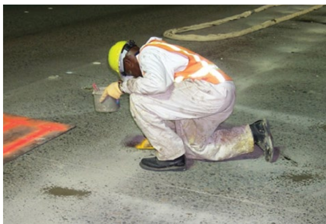
Figure 4.8. Patching drill holes
