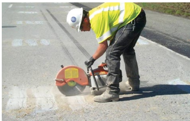
Figure 8.22. Sawcutting to reestablish the transverse joint through the patching material
