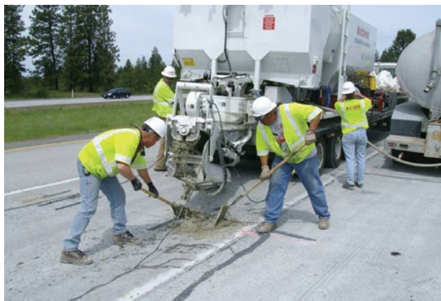
Figure 8.20. Placing patching material into dowel bar slots
