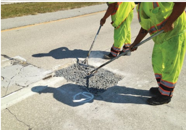
Figure 5.22. Placement of proprietary polymer-based repair material with premixed aggregates
