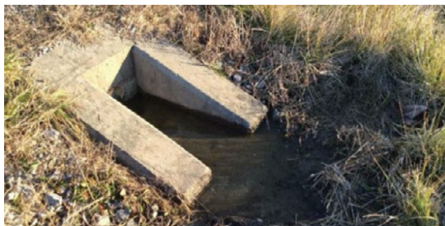
Figure 7.10. Edgedrain outlet pipe holding water due to inadequate ditch grade
