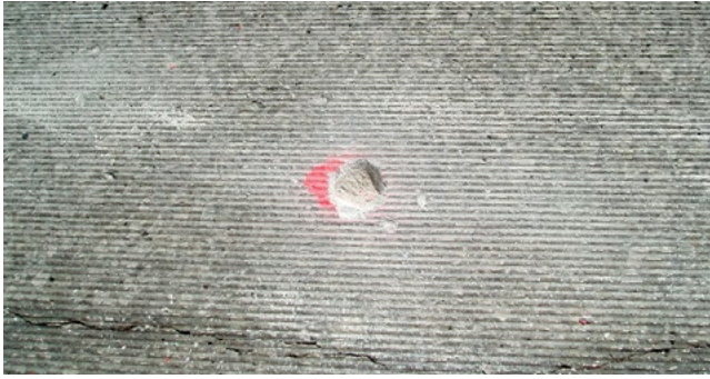
Figure 8.25. Pilot hole drilled in slab
