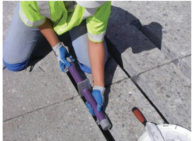
Figure 8.18. Placing a dowel bar assembly into a slot
