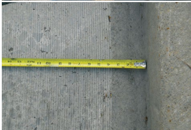
Figure 9.11. Gutter apron before (top) and after (bottom) a feathering pass
