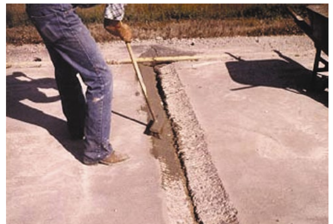
Figure 5.23. Application of cement grout as bonding agent
