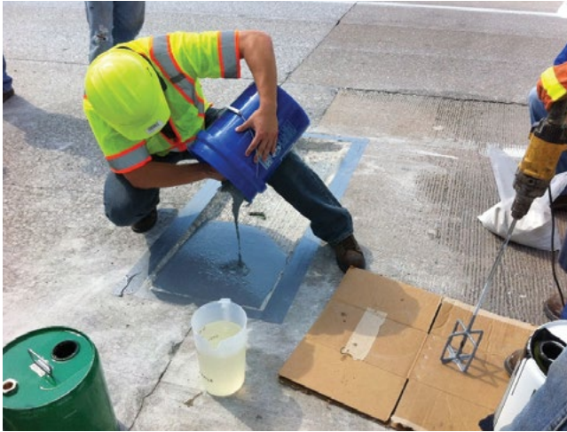
Figure 5.21. Placement of proprietary polymer-based repair material without aggregates
