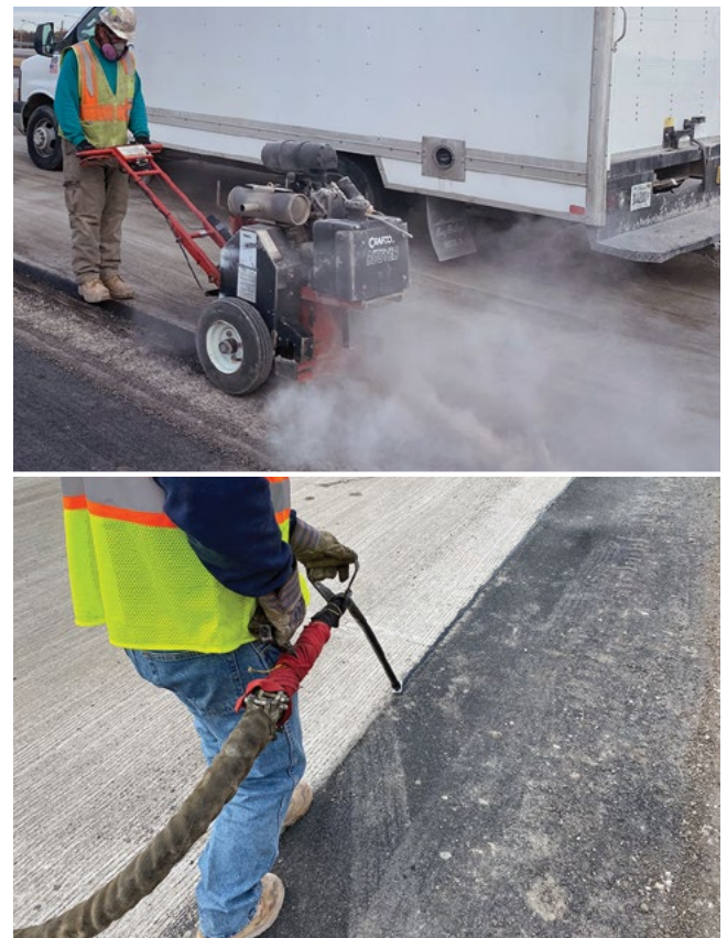
Figure 10.19. Routing (top) and sealing (bottom) of a longitudinal joint between a concrete mainline and asphalt shoulder
