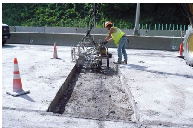
Figure 6.17. Example of a gang drill used for dowel bar installation
