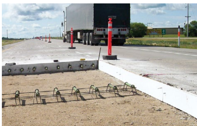
Figure 6.7. Bond breaker along longitudinal lane-lane joint
