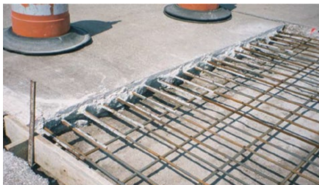
Figure 6.23. CRCP repair with both longitudinal and transverse steel
