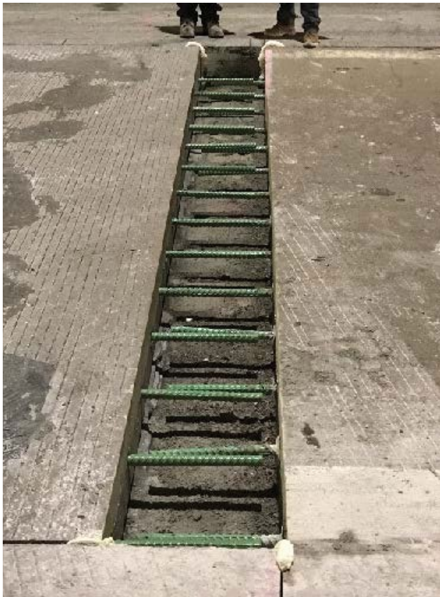
Figure 6.11. Splice zone between new precast panel and existing CRCP
