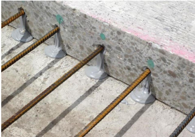
Figure 6.9. TxDOT method of CRCP repair
