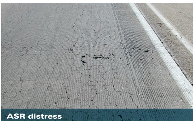
Figure 3.1. Common concrete pavement distress types
