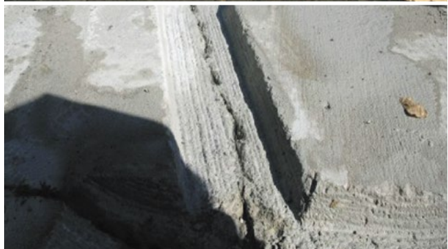
Figure 5.16. Vertical edge mill head (top) and milling pattern (bottom)
