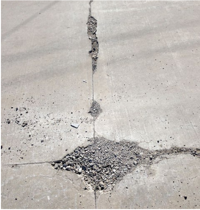
Figure 10.2. Joint deterioration of concrete pavement
