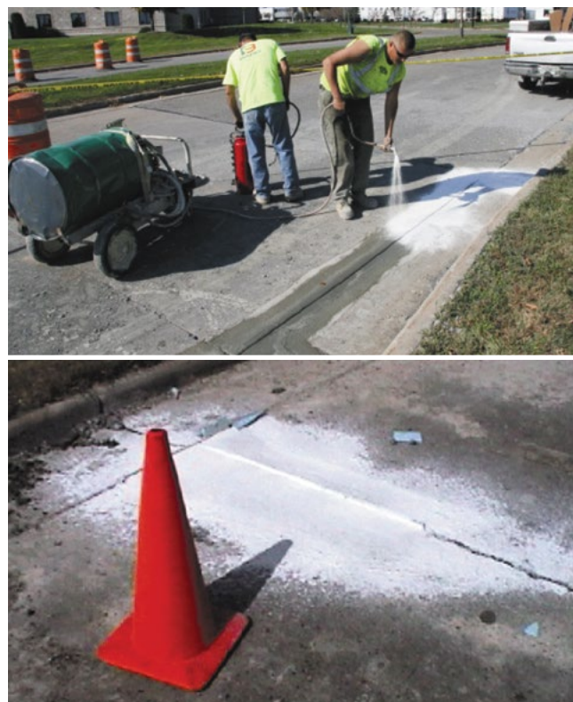
Figure 5.28. PDR material curing operations
