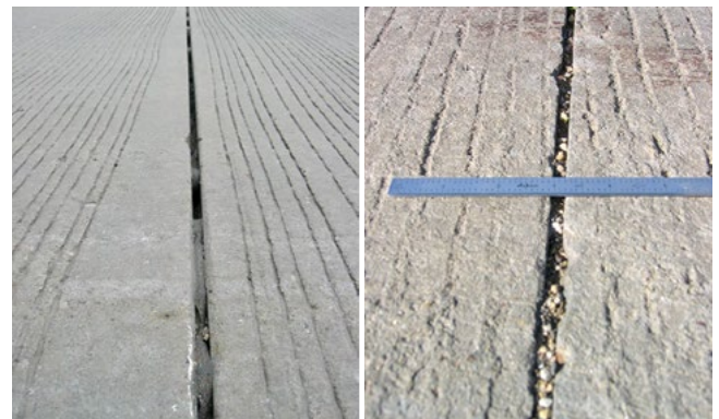
Figure 10.4. Examples of joint sealant failures: missing and debonded sealant (left) and incompressible materials in joint (right)
