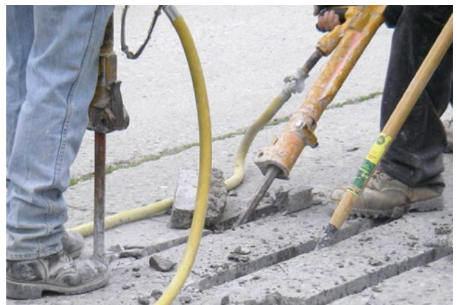
Figure 8.12. Operating jackhammers at no more than a 45-degree angle
