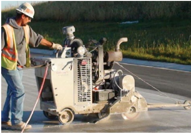
Figure 10.11. Sealant removal through joint sawing
