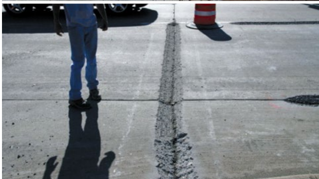
Figure 5.14. V-shaped milling head (top) and milling pattern (bottom)
