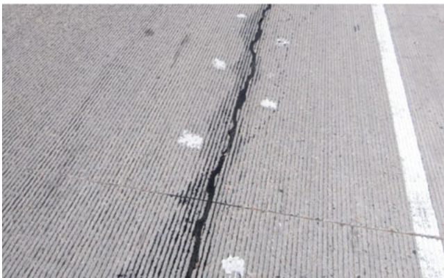
Figure 8.28. Completed cross-stitching
