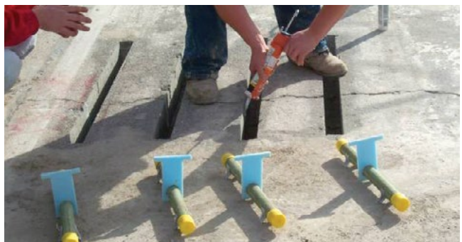
Figure 8.15. Media-blasted and cleaned slot
