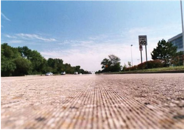
Figure 9.2. Surface texture provided by diamond grinding
