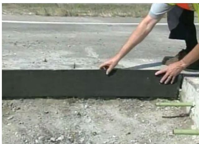
Figure 6.24. Placing a bond breaker board along a longitudinal lane-lane joint
