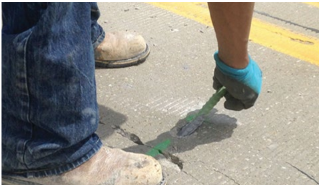
Figure 8.27. Inserting a tie bar into a drilled hole
