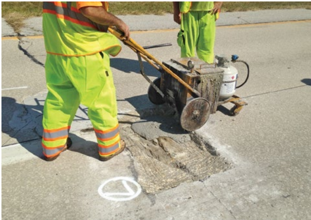
Figure 5.21. Placement of proprietary polymer-based repair material without aggregates
