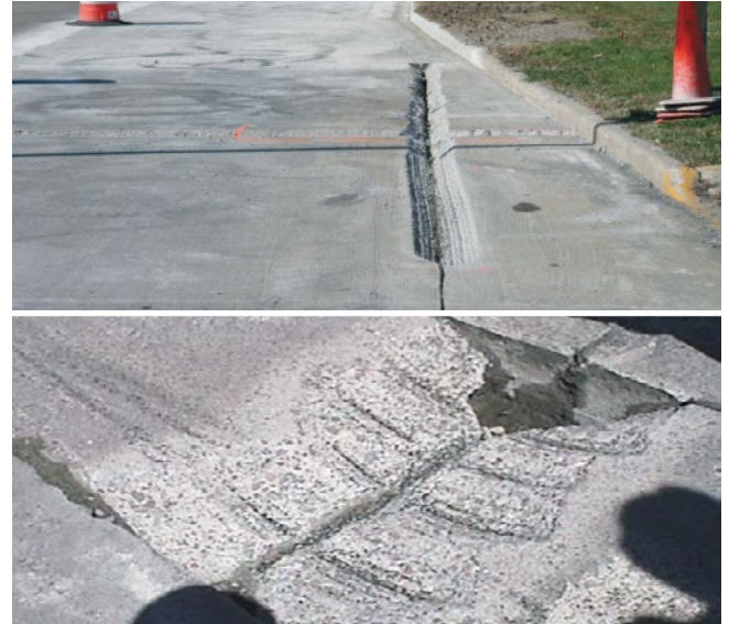
Figure 5.13. Milling options: milling along a joint (top) and dish-shaped milling perpendicular to a joint (bottom)
