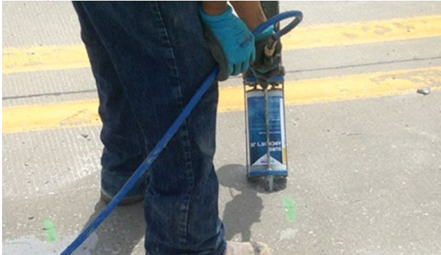
Figure 8.26. Injecting epoxy into a drilled hole used for cross-stitching
