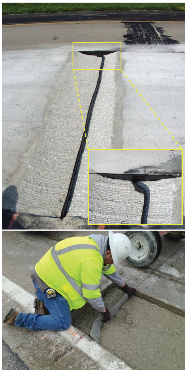
Figure 5.20. Placement of bond breaker on a PDR project
