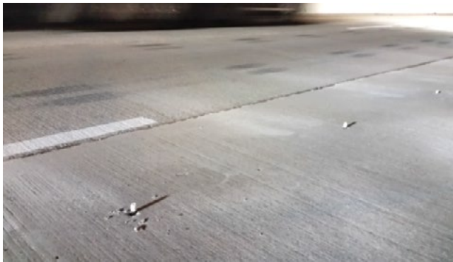
Figure 4.18. Injection holes in concrete slab
