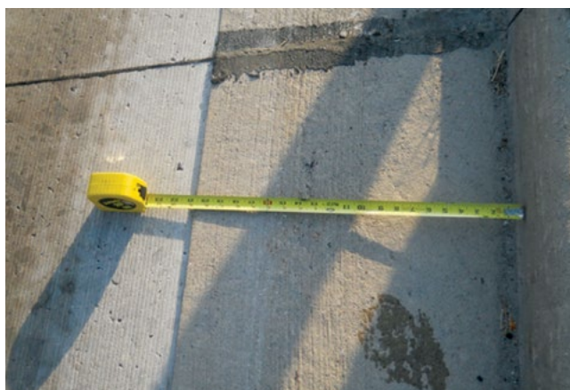
Figure 9.10. Holiday on a diamond-ground surface
