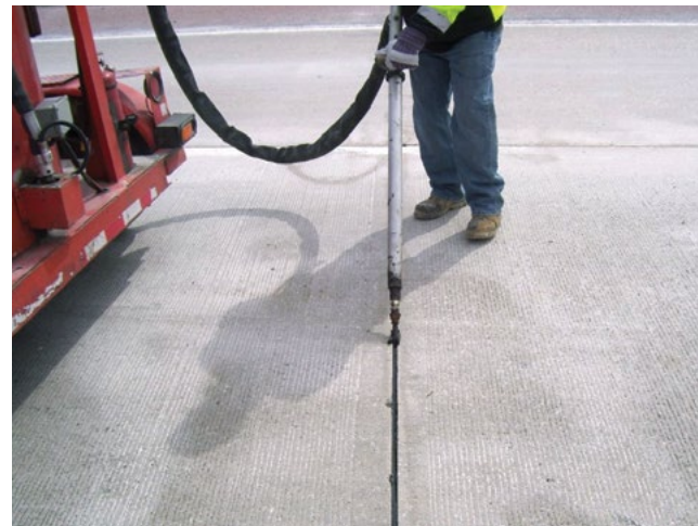
Figure 10.15. Installation of hot-applied asphalt joint sealant
