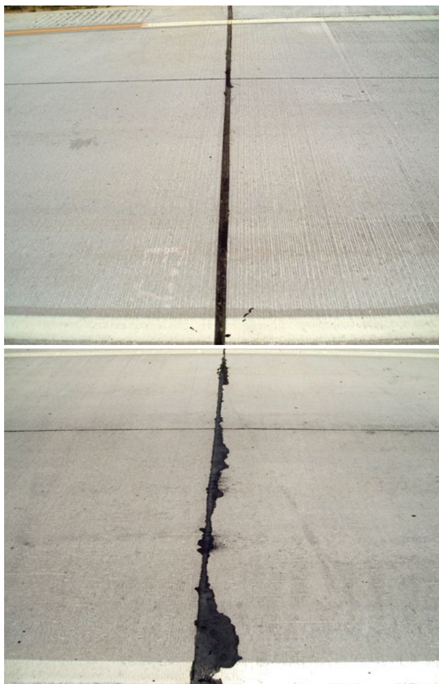
Figure 10.17. New expansion joint (top) and older expansion joint with extruded sealant shoulder (bottom)
