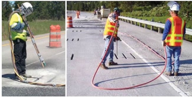
Figure 8.14. Media blasting to remove residue (left) and air blasting immediately prior to dowel placement (right)
