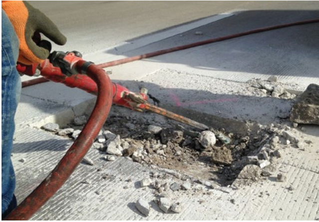
Figure 5.12. Repair area prepared using the chip-and-patch (Type 1) procedure
