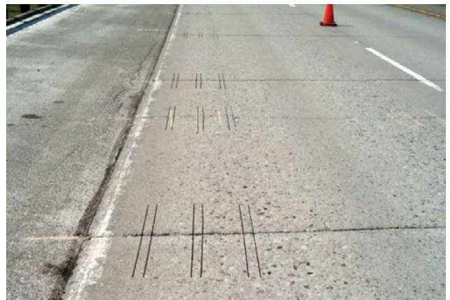
Figure 8.11. Sawcuts for dowel bar slots across transverse joints
