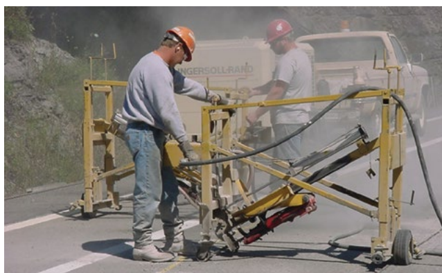
Figure 8.24. Drilling holes for cross-stitching
