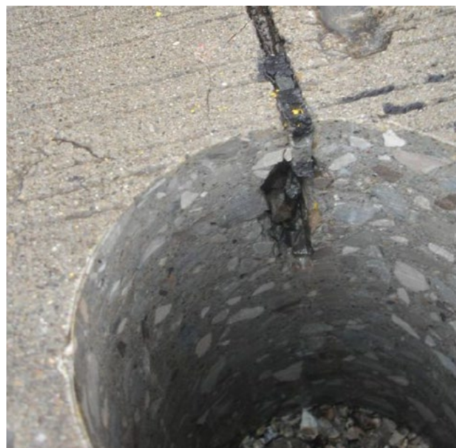
Figure 10.9. Deterioration below the joint sealant
