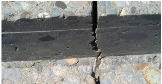
Figure 8.15. Media-blasted and cleaned slot
