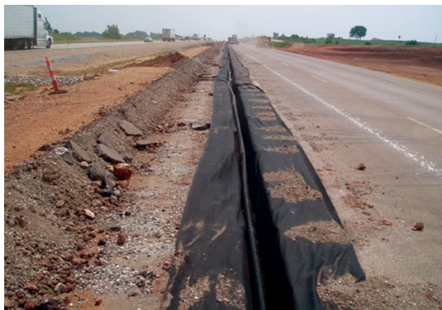
Figure 7.13. Geotextile-lined trench with CPE pipe
