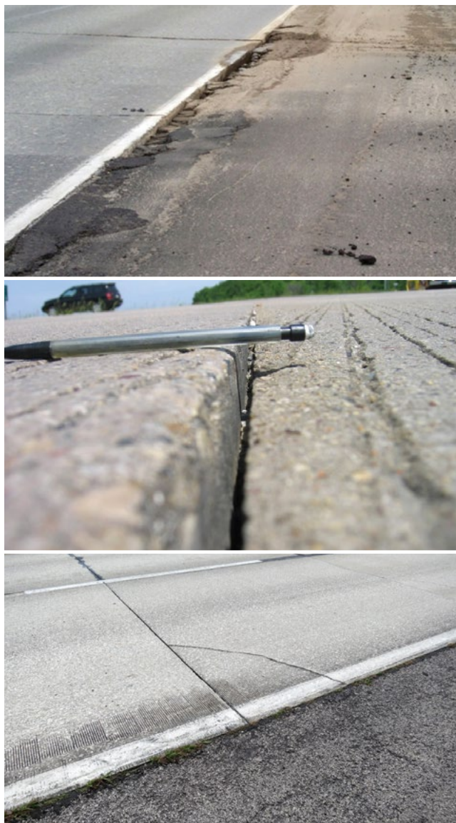
Figure 10.1. Pumping (top), faulting (center), and corner break (bottom) distresses
