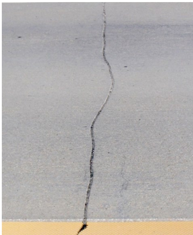
Figure 10.20. Sealed transverse crack
