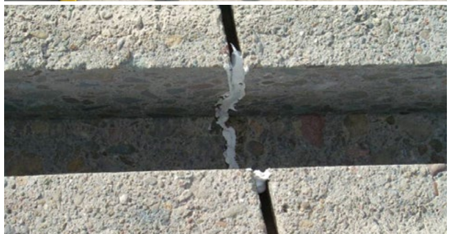
Figure 8.16. Applying caulk to dowel bar slot sides and bottom (top) and caulked pavement joint (bottom)
