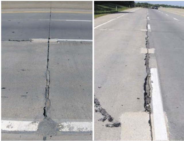
Figure 5.3. Candidate distresses for Type 2 PDRs
