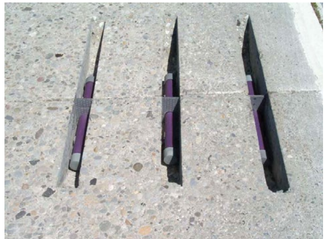
Figure 8.19. Dowel bars placed in slots
