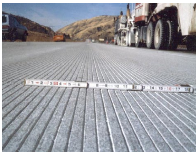
Figure 9.13. Longitudinally diamond-grooved surface
