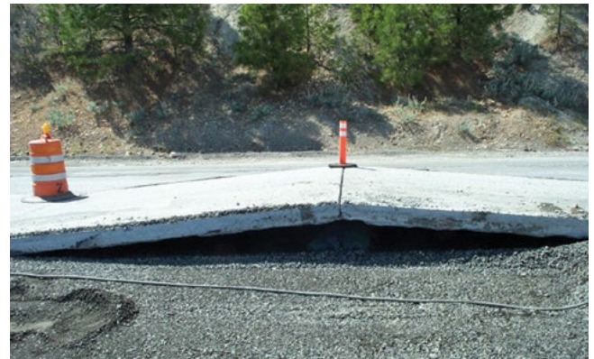
Figure 10.3. Concrete pavement joint spalling (top) and blowup (bottom)
