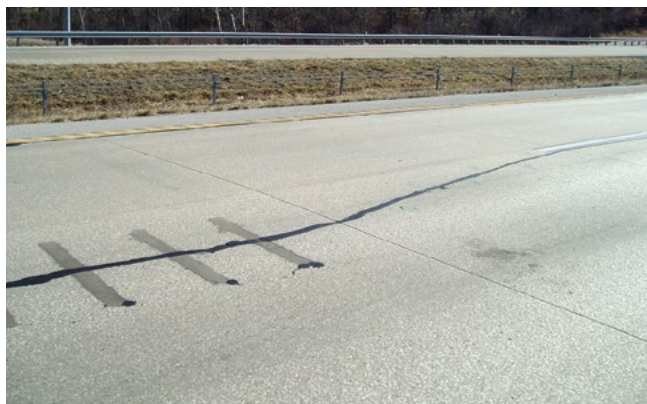
Figure 8.30. Completed slot-stitching of a longitudinal crack
