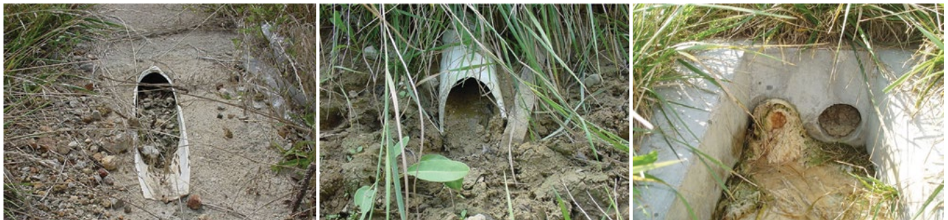
Figure 7.19. Clogged edgedrain outlet pipes
