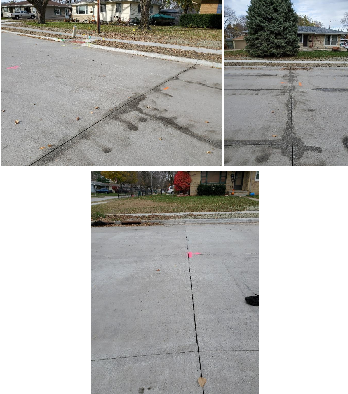
Figure 27. Landmarks showing western edge of SoTA application (top left), mid-point where sealers were switched (top right), and eastern edge of 40% silane application (bottom)
