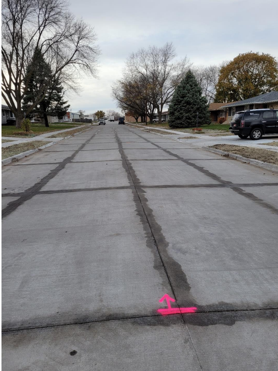
Figure 26. Sealer application on SE 8th Street
