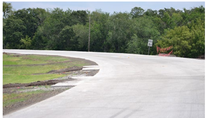
ACPA, used with permission (Duit Construction Company, Inc.)
