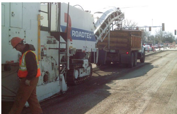
Figure 28. Partial-depth milling of the existing asphalt overlay(s), with the asphalt remaining after milling utilized as a separation layer for the unbonded concrete overlay
