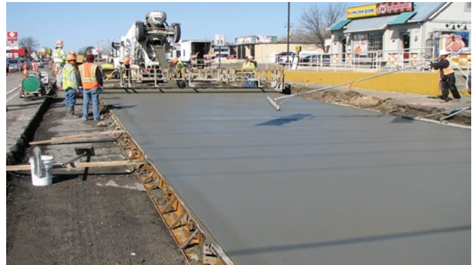
Figure 29. Traditional fixed-form methods being used to construct the unbonded concrete overlay
