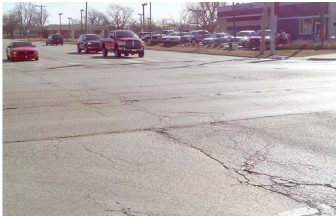
Figure 27. Existing pavement condition prior to placement of the unbonded concrete overlay
