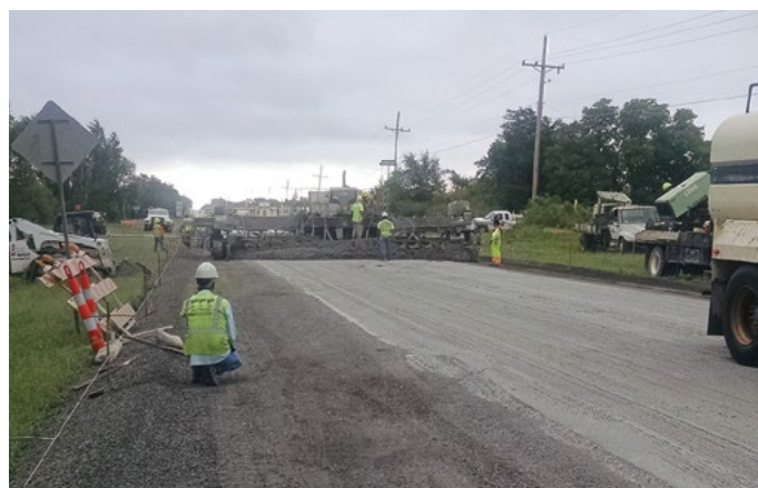
ACPA, used with permission (Duit Construction Company, Inc.)
