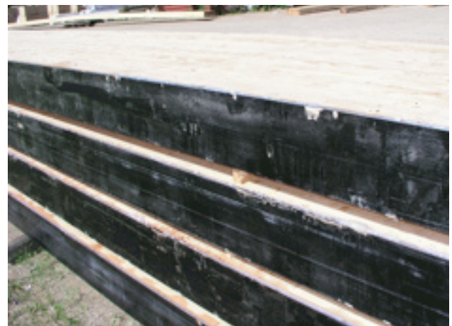
Glued-laminated girders after FRP installation
