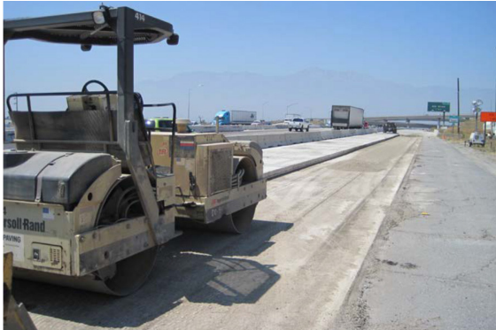
I-15 near Ontario, California, CTB layer after removal of pavement
