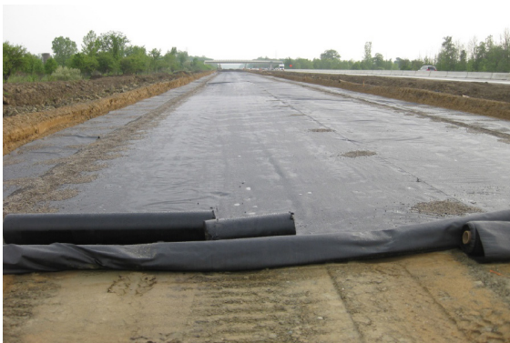
I-94 in St. Clair and Macomb Counties, Michigan, woven geotextile separator installed on top of the subgrade
