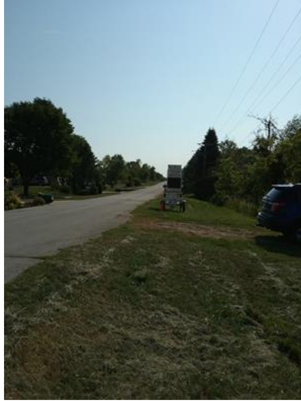
Figure 4-15. NE 134th Avenue West site trailer setup
