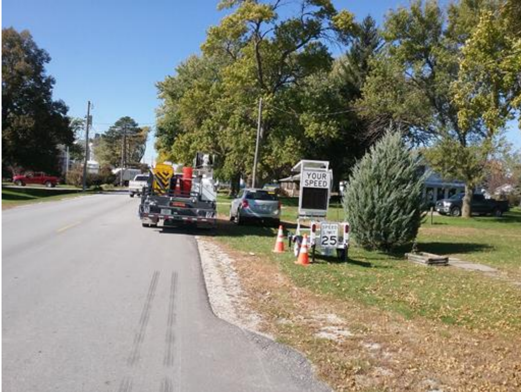
Figure 4-2. County Highway F50 trailer setup
