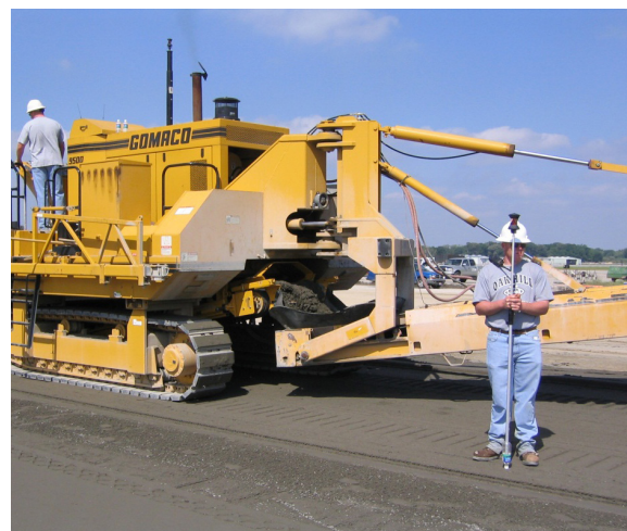
Figure 11. Checking finished elevations behind the paving machine. Courtesy ACPA 2013
