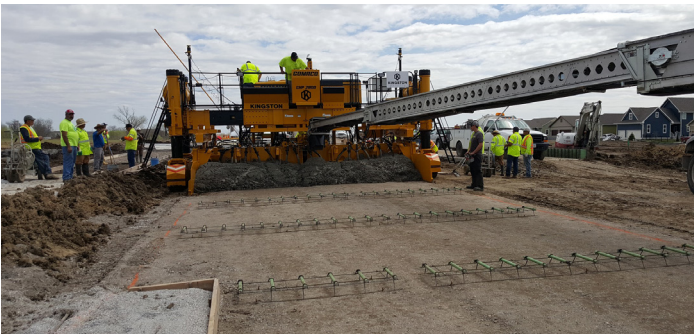
Figure 9. A paving machine utilizing laser-augmented GPS. Photo courtesy: Snyder & Associates, Inc.
