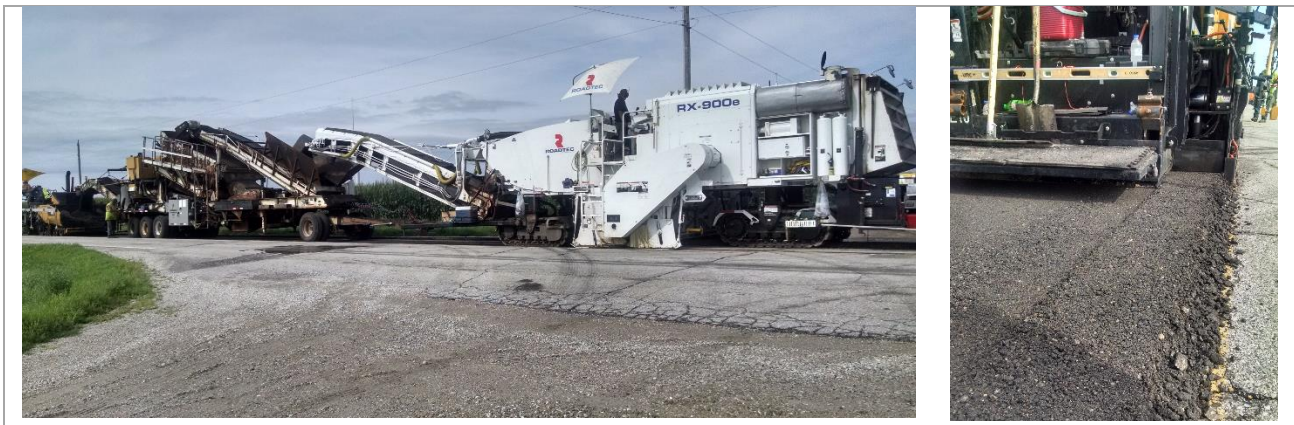
Figure 9. CIR operations: train, left, and pavement placement, right
