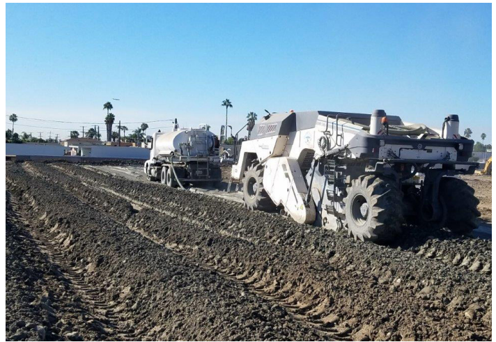
Figure 13. Mixing cement and subgrade (©2020 Pavement Recycling Systems, Inc., used with permission)
