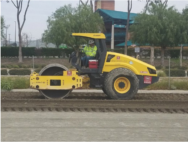
Figure 10. Smooth drum roller (©2020 Pavement Recycling Systems, Inc., used with permission)
