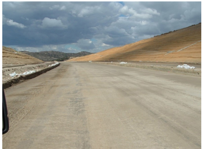
Figure 12. Compacted subgrade ((Jeff Wykoff, California Nevada Cement Association, used with permission)
