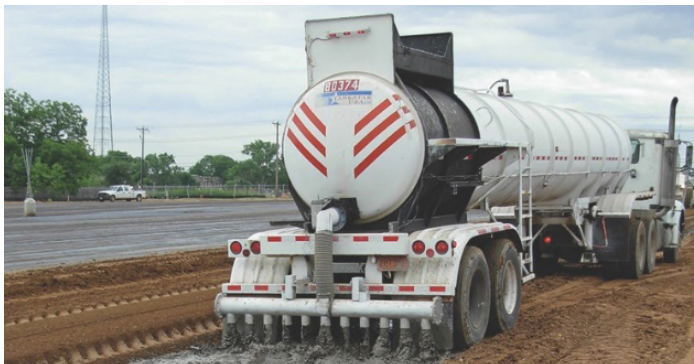
Figure 6. Spreading portland cement slurry (Halsted et al. 2008, ©2008 PCA, used with permission)
