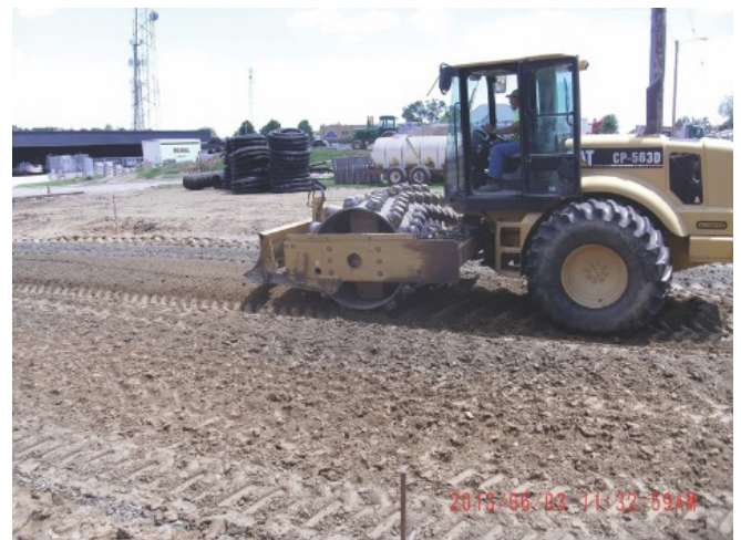
Figure 9. Vibratory sheepsfoot tamping roller (©2020 Pavement Recycling Systems, Inc., used with permission)
