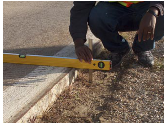
Measuring pavement edge drop-off
