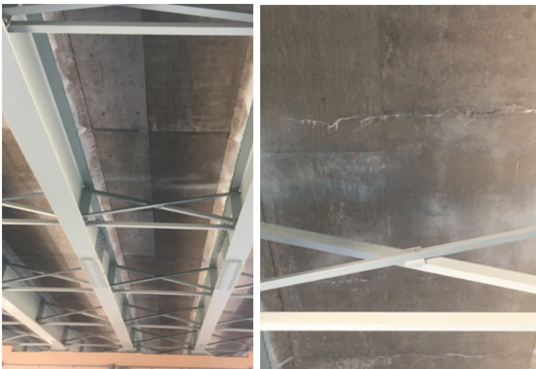
Figure 12. I-271 NB (internally cured deck) and I-271 SB (normal concrete deck)
