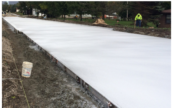
Figure 6. Proper curing compound application
