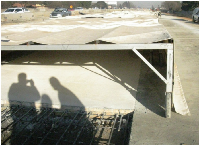
Figure 4. A rolling tent structure
