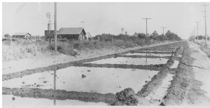
Figure 2. Flooding of an Iowa roadway (photo courtesy of Mitchell County, Iowa)
