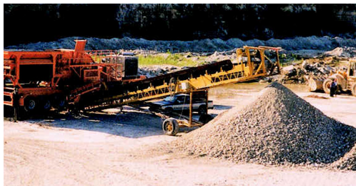
Figure 6. Typical concrete pavement recycling crushing and stockpiling operation
