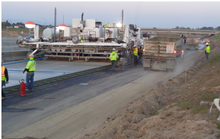
Figure 7. Paving on I-84 in Boise, Idaho
