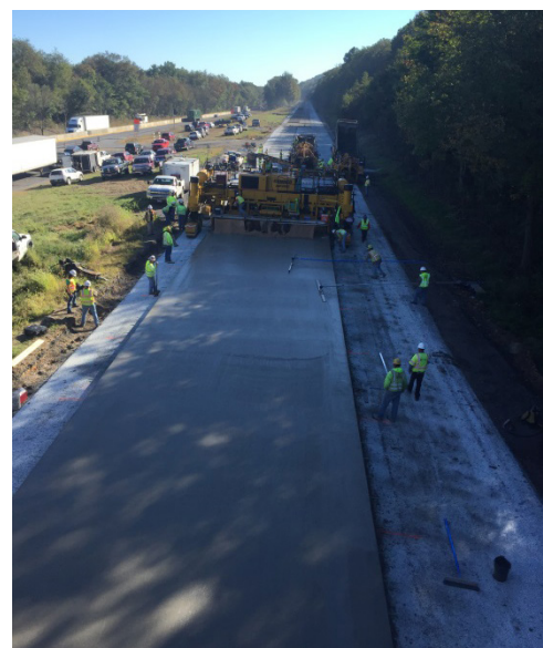
Figure 4. Paving on I-81 in central Pennsylvania
