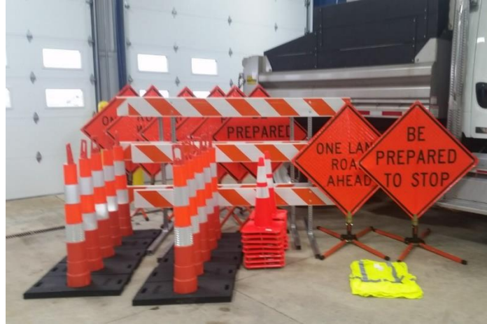
Figure 1. Work zone sign package
