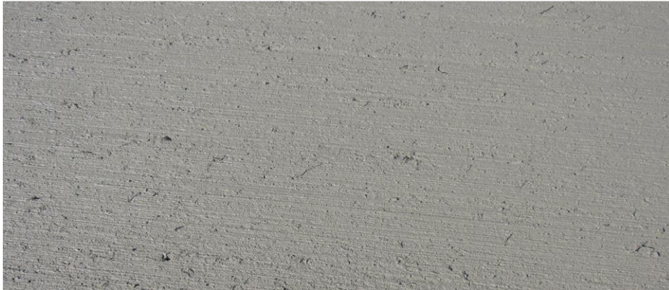
Figure 6.3. FRC overlay with 4 lb/yd 3 of synthetic macrofiber showing excellent finishability
