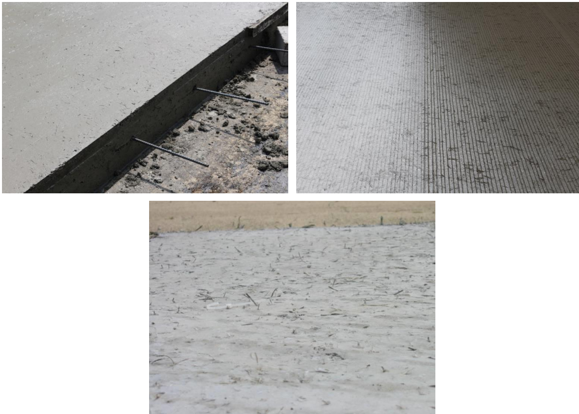
Figure 6.2. Examples of the surface appearance of FRC with a slipform pavement edge (upper left), with the use of transverse tining and curing compound (upper right), and for a hand-finished troweled surface (bottom)
