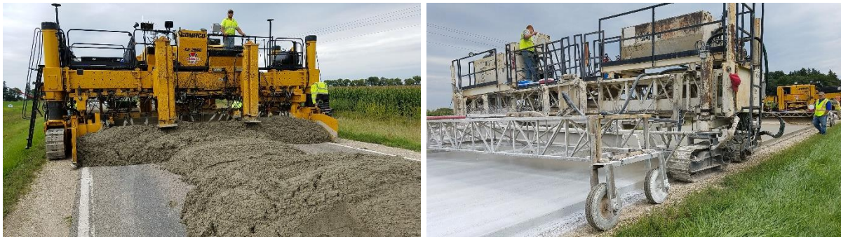
Figure 6.1. Construction of an FRC overlay in Iowa
