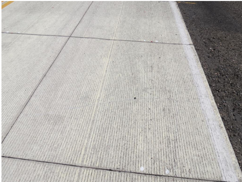
Figure 6.4. FRC overlays with synthetic macrofibers and longitudinal tining
