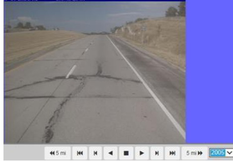
(a) Pre-existing condition (2005)
