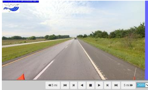
(b) Condition just after paving in 2009
