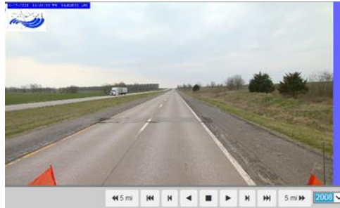
(a) Pre-existing condition (2008)
