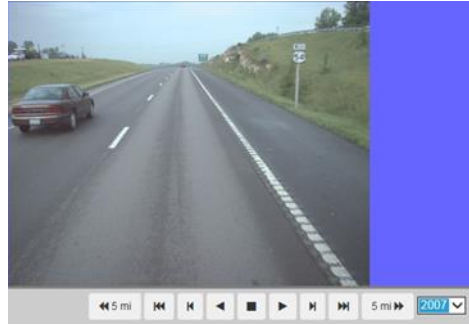
(b) Condition just after paving in 2007
