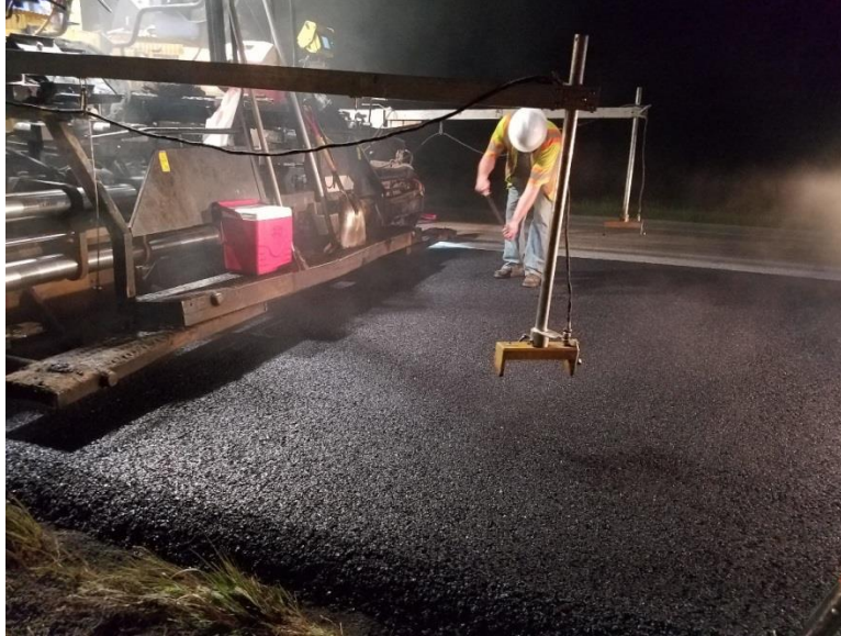
Figure 6-4. ECR SMA night paving on I-35 mainline in spring 2018
