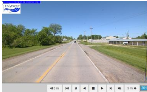
(b) Condition just after paving in 2010
