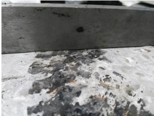
Figure 4.10. Rut depth of a CCAM slab
