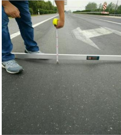
(a) Asphalt pavement
