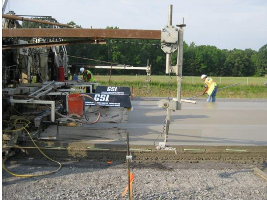
Figure 21. Paver-mounted GSI setup on paver with OCB
