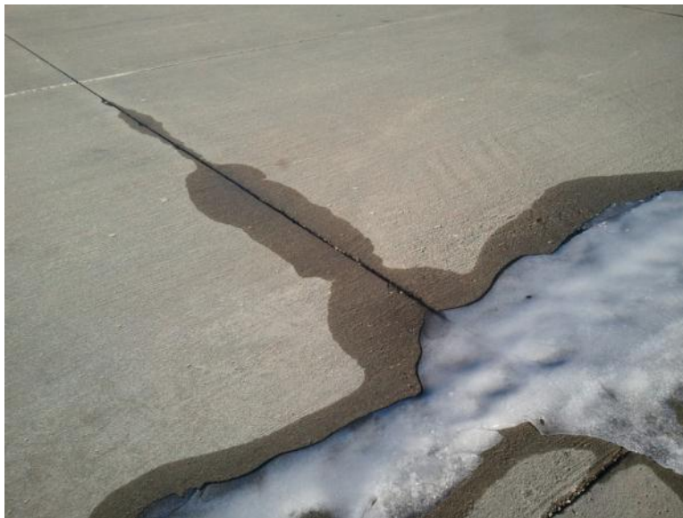
Figure 18. Illustration of local differences in moisture state in a single slab
