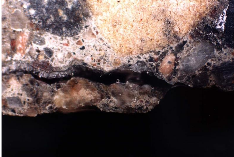
Figure 6. Salt deposits inside a crack
