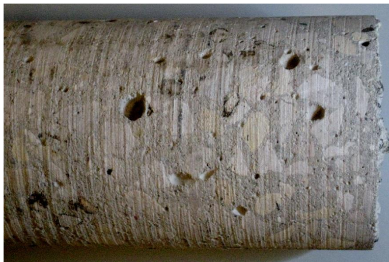
Figure 21. A core with large air voids (Is it sufficiently consolidated?)
