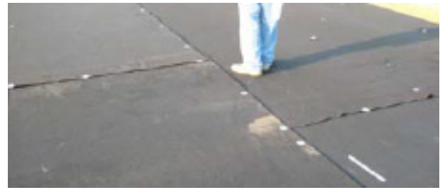
Figure 5. Overlap of nonwoven geotextile material section
