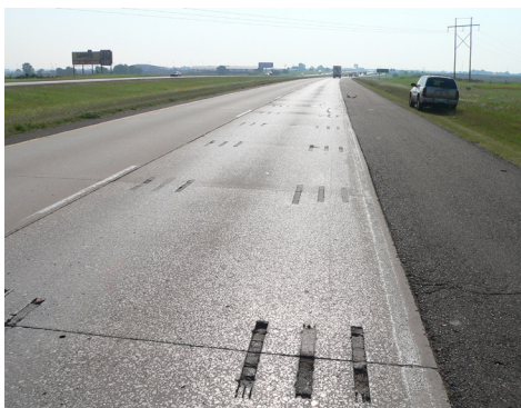
a) I-40 before overlay placement
