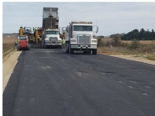
Figure 1. Placement of nonwoven geotextile interlayer
