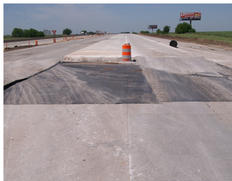
b) I-40 after overlay placement (2009-2010)
