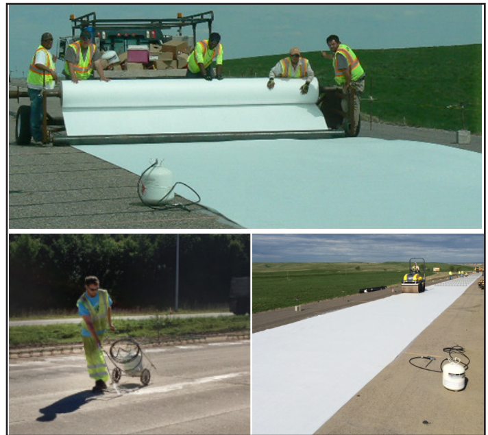
Figure 7. Securing geotextile with spray adhesive
