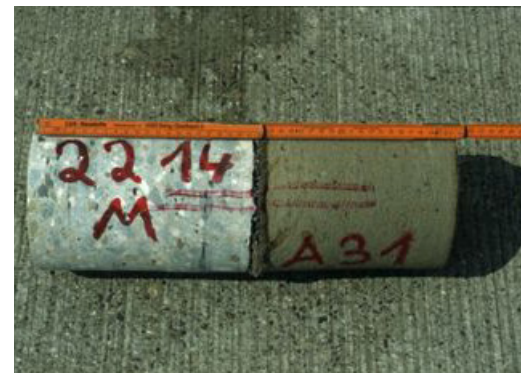
Figure 2. Core from Germany showing nonwoven geotextile interlayer between surface concrete (left) and cement-treated base (right)
