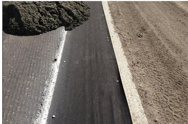
**Figure 32. Non-woven geotextile placed over concrete in unbonded overlay**
