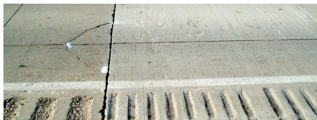
Figure 21. Interior corner cracking
