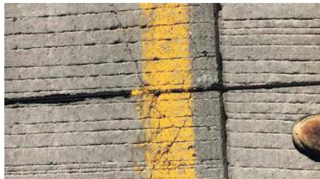
**Figure 23. Restraint cracking**
