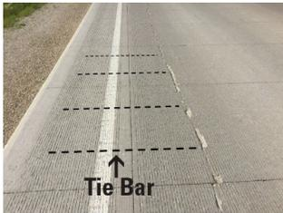
Figure 11. Longitudinal cracking along end of tie bar
