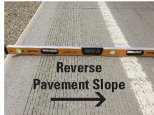
Figure 12. Improper cross-slope from heave
