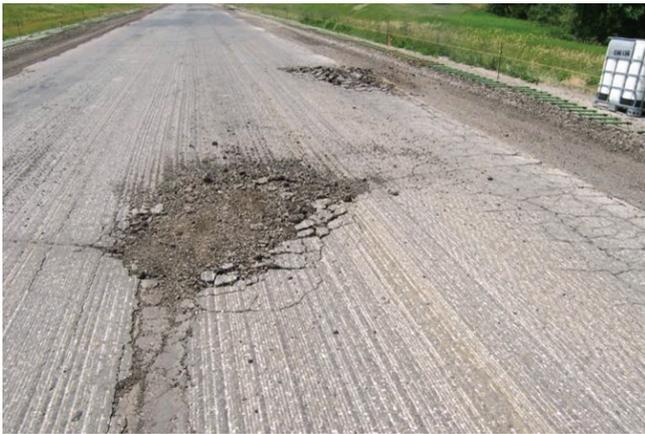
**Figure 31. Construction equipment hauling damage of remaining asphalt after milling**
