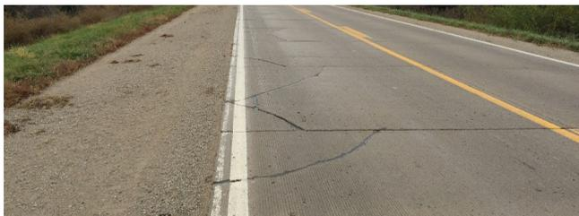
**Figure 22. Exterior corner cracking**
