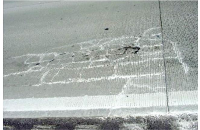
**Figure 29. Cracking from joint lockup**
