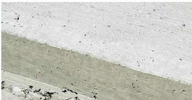
Figure 26. Concrete overlay with synthetic fibers
