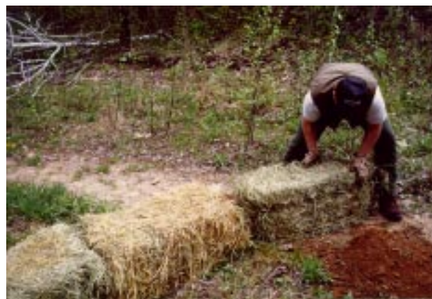
Figure 8.— Installation of hay or straw bale barriers.
