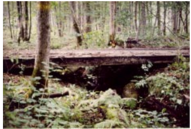
Figure 22.— Temporary bridge spanning a stream.
