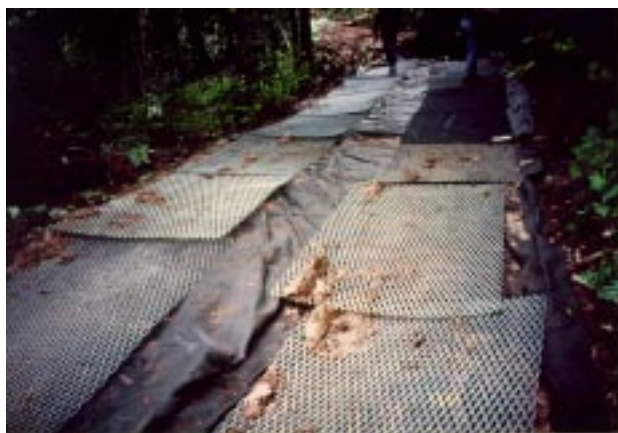
Figure 37.— Expanded metal grating over a geotextile.
