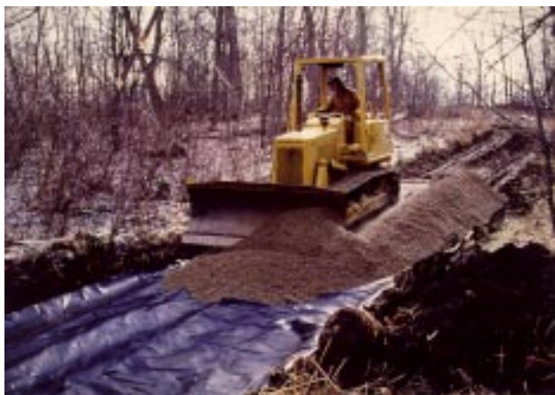
Figure 15.—A geotextile used in a ford.
