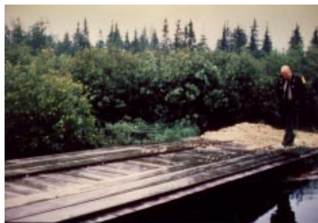
Figure 28.—Bridge made from a used railroad car.
