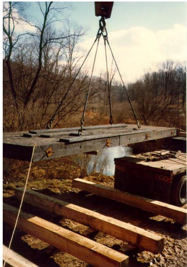
Figure 27.—Stress-laminated timber bridge panel.
