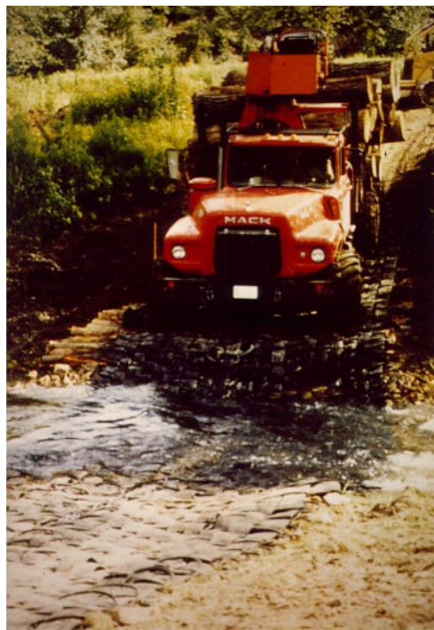
Figure 16.—A tire mat used to provide support in a temporary ford.
