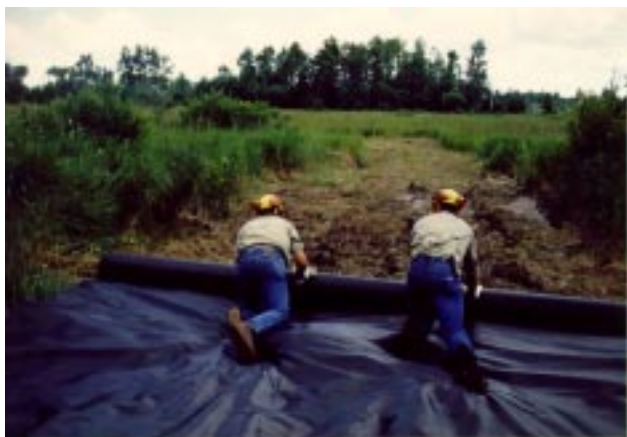
Figure 32.—Applying a geotextile under a temporary wetland crossing.
