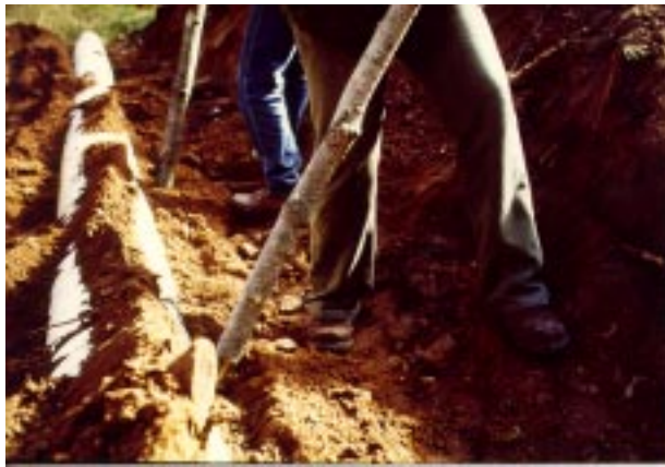
Figure 18.— Packing earth around a culvert during installation.
