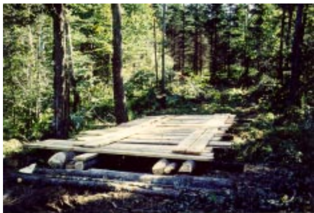
Figure 5.—Abutment logs below a log stringer bridge (approach yet to be constructed).
