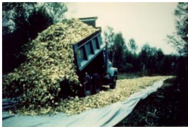
Figure 46.—Use of a geotextile under wood aggregate.
