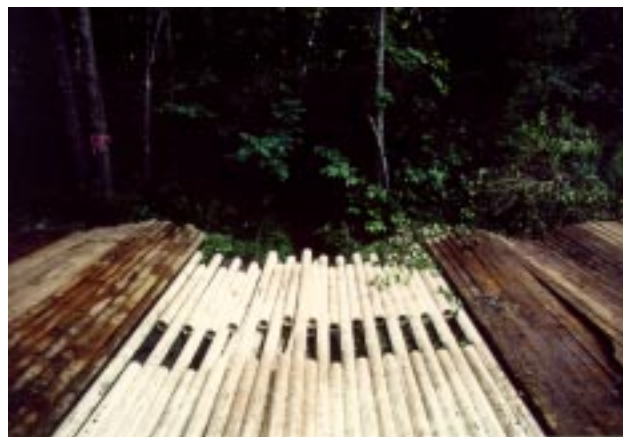
Figure 38.— PVC or HDPE pipe mat in a road.
