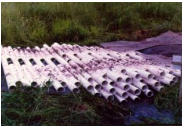
Figure 21.—Pipe bundle crossing layered to the desired height.
