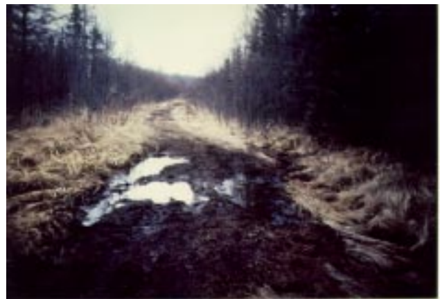
Figure 31.— Wet area in a haul road.
