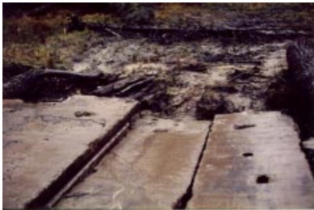
Figure 30.— Pre-stressed concrete bridge.
