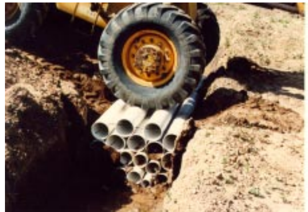
Figure 19.— PVC or HDPE pipe bundle.
