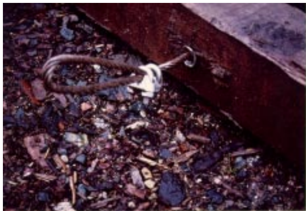
Figure 34.—Cable loop at the end of a wood mat.
