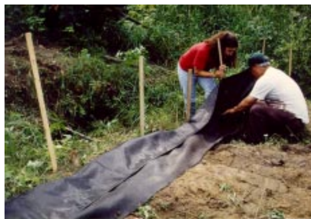
Figure 9.— Installation of silt fencing.
