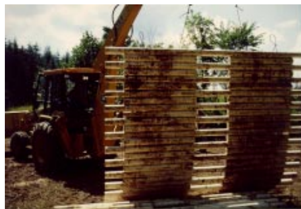
Figure 39.— PVC or HDPE pipe mat.
