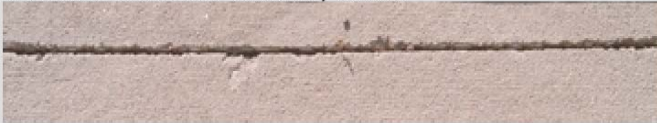
B. MODERATE RAVELING – Sawn early in window
