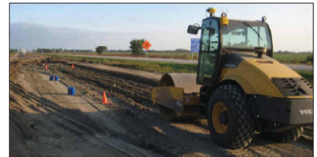
Figure 1. Smooth-drum roller equipped with onboard display unit
