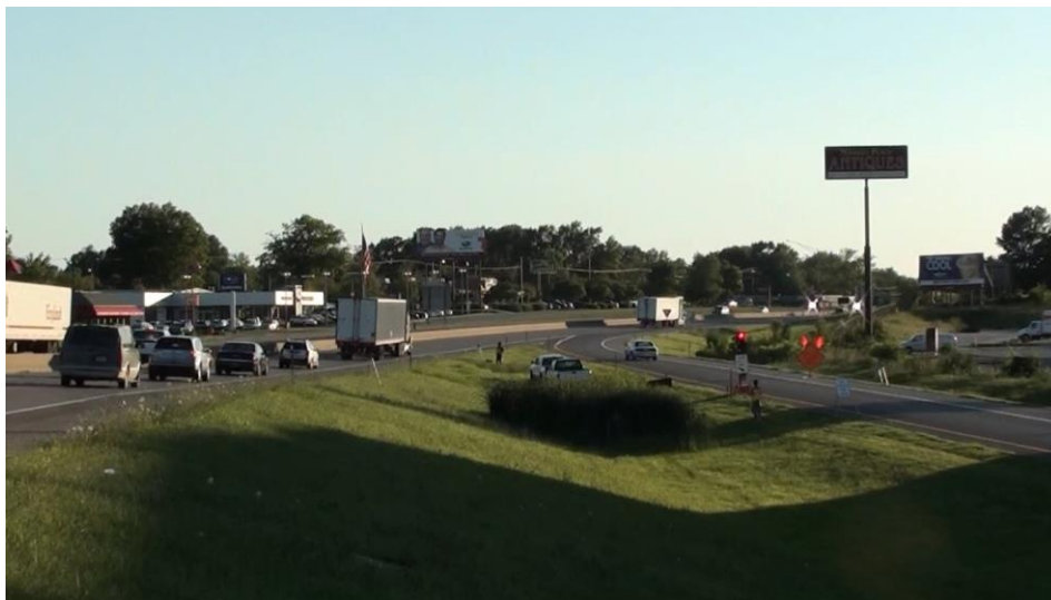
Figure 1 Temporary ramp meter near a work zone.
