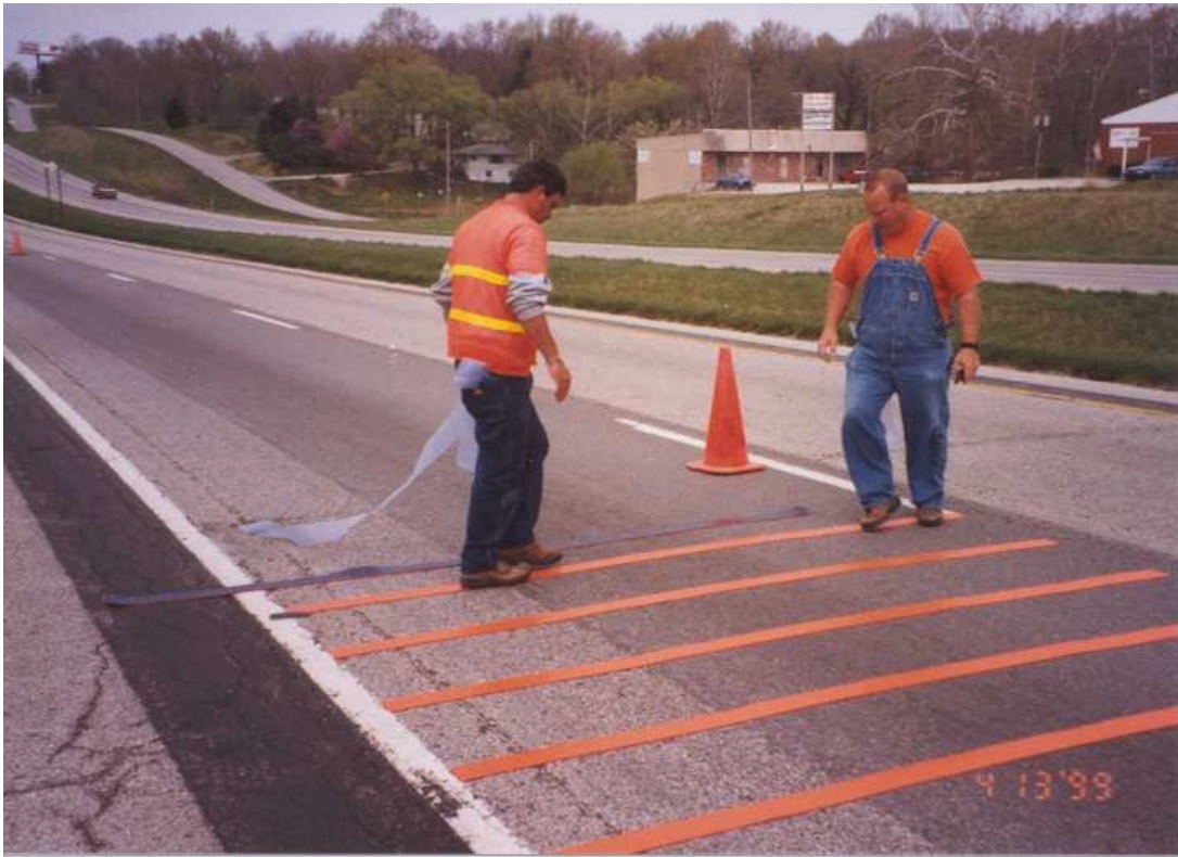
FIGURE 4-15 Rumble strips initial installation.
