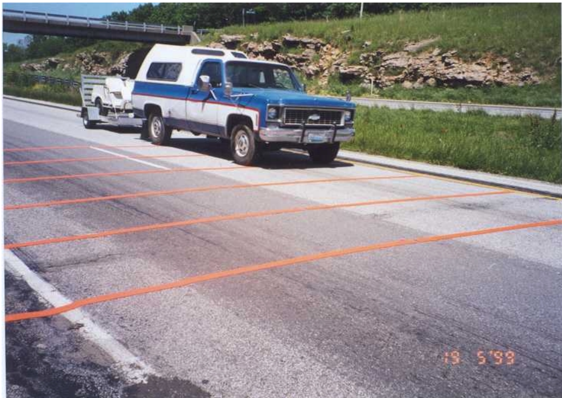
FIGURE 4-4 Rumble strips on 5' centers.
