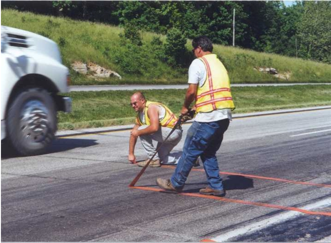
FIGURE 4-20 Rumble strip removal.
