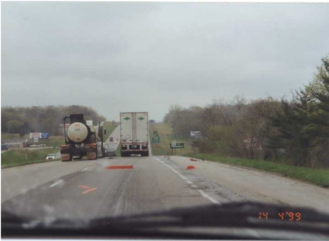
FIGURE 4-17 Failure of rumble strips when improperly installed.
