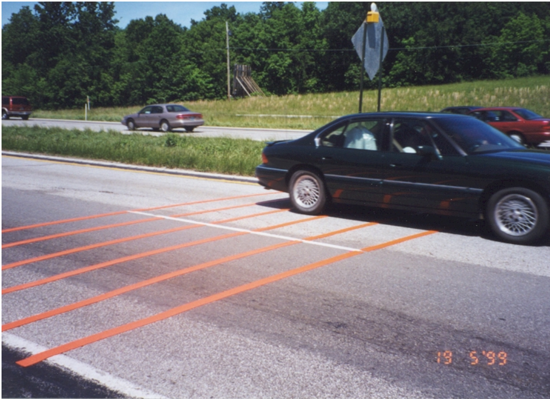
FIGURE 4-5 Rumble strips on 2' centers.
