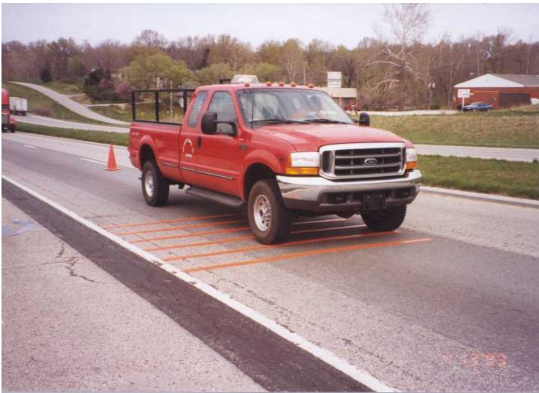
FIGURE 4-16 Rumble strips initial installation.
