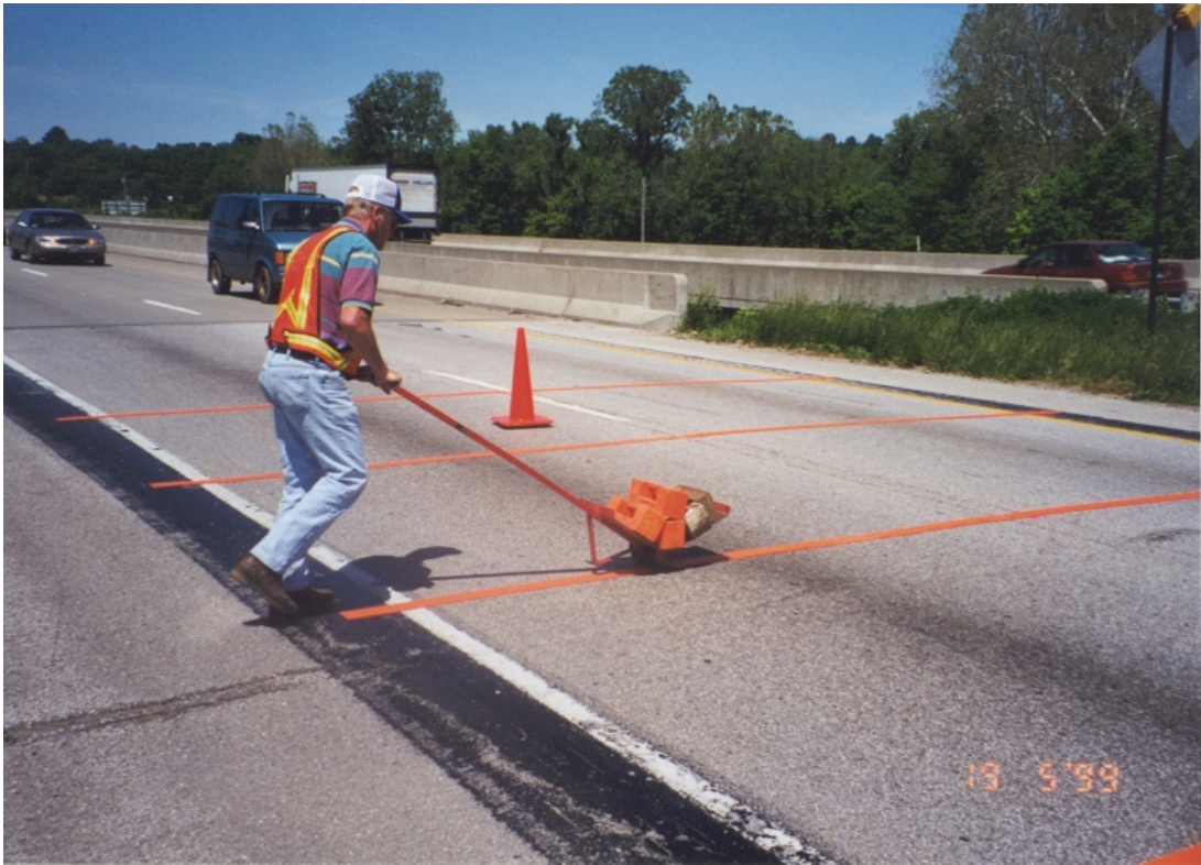
FIGURE 4-3 Installation of rumble strips on 10' centers with 200-lb roller.
