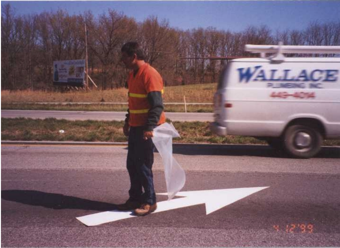
Figure 4-35 Arrow installation.
