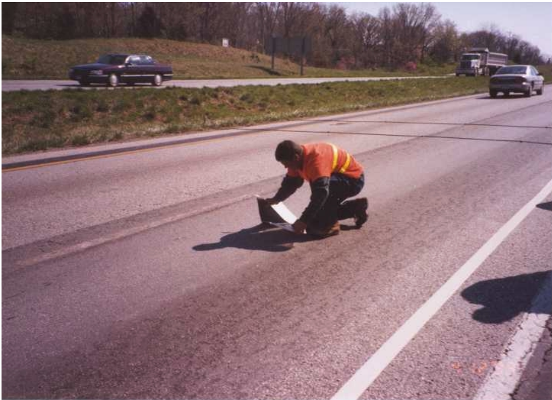
Figure 4-34 Arrow installation.
