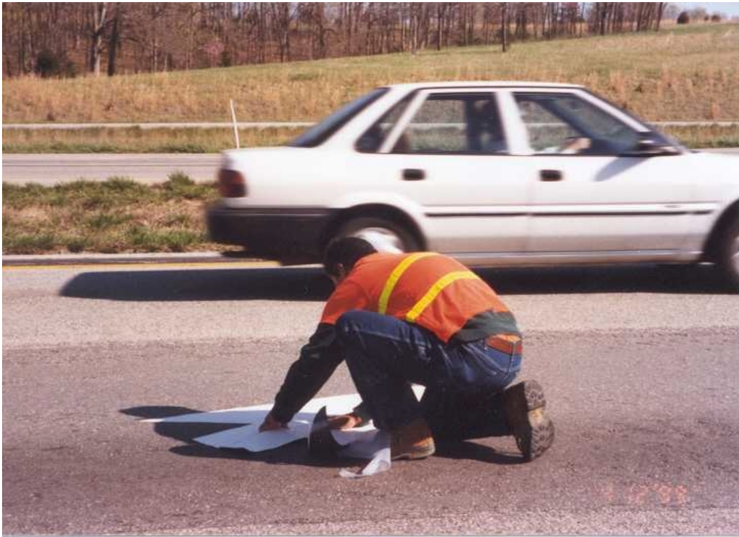
Figure 4-33 Arrow installation.
