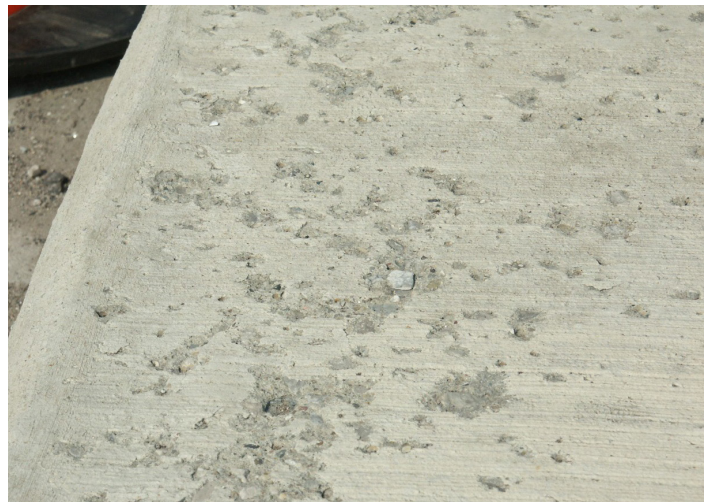
Figure 5b. Example of flaking
