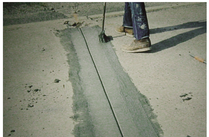
Figure 9. Edge sealing using sand-cement grout after placement of patch material
