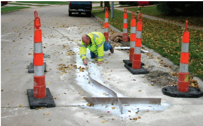
Figure 7. Cutting excess compressible material used as bond breaker in longitudinal crack
