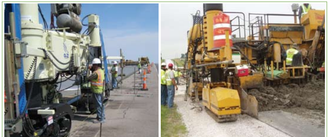
Figure 1: Stringline (left) and stringless (right) pavers
