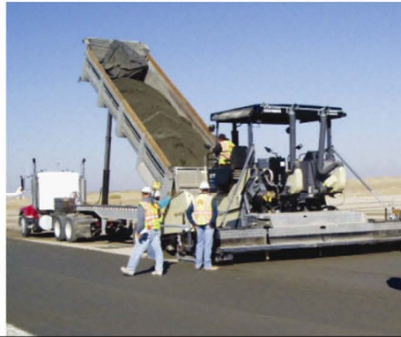
Figure 3. RCC combines aspects of conventional concrete pavement with construction practices similar to HMA pavement.
