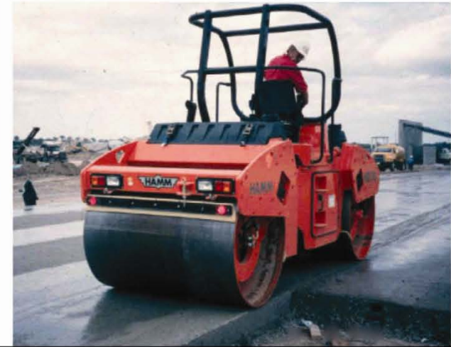
Figure 3. RCC combines aspects of conventional concrete pavement with construction practices similar to HMA pavement.
