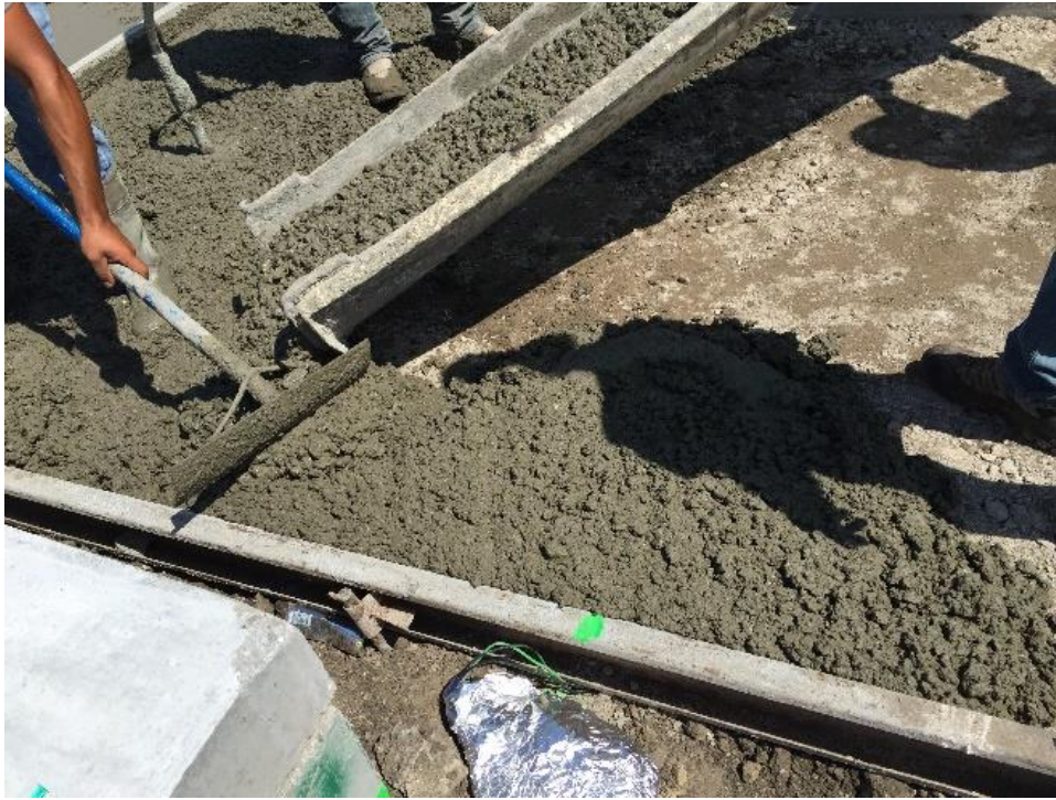
Figure 3. Placing concrete and embedding sensors
