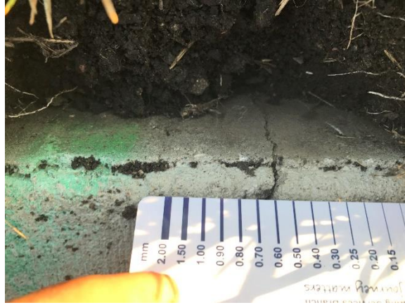
Figure 55. Joint 6 in the control section
