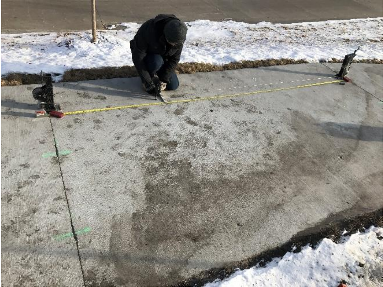
Figure 16. Portable device for measuring deflection over time
