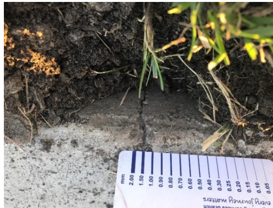
Figure 50. Joint 1 in the control section
