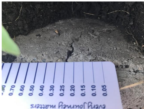
Figure 54. Joint 5 in the control section
