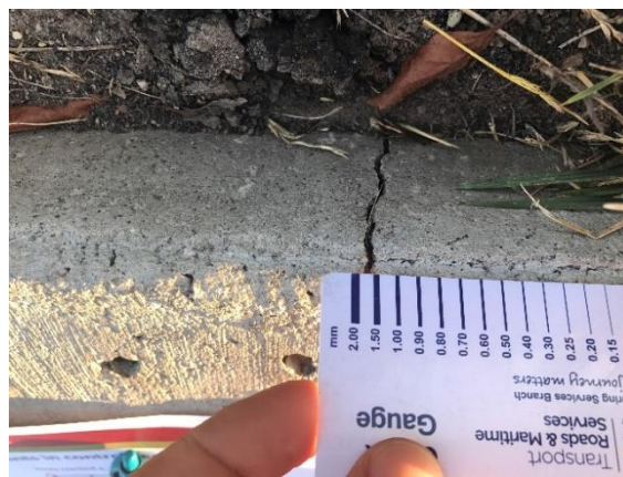
Figure 51. Joint 2 in the control section
