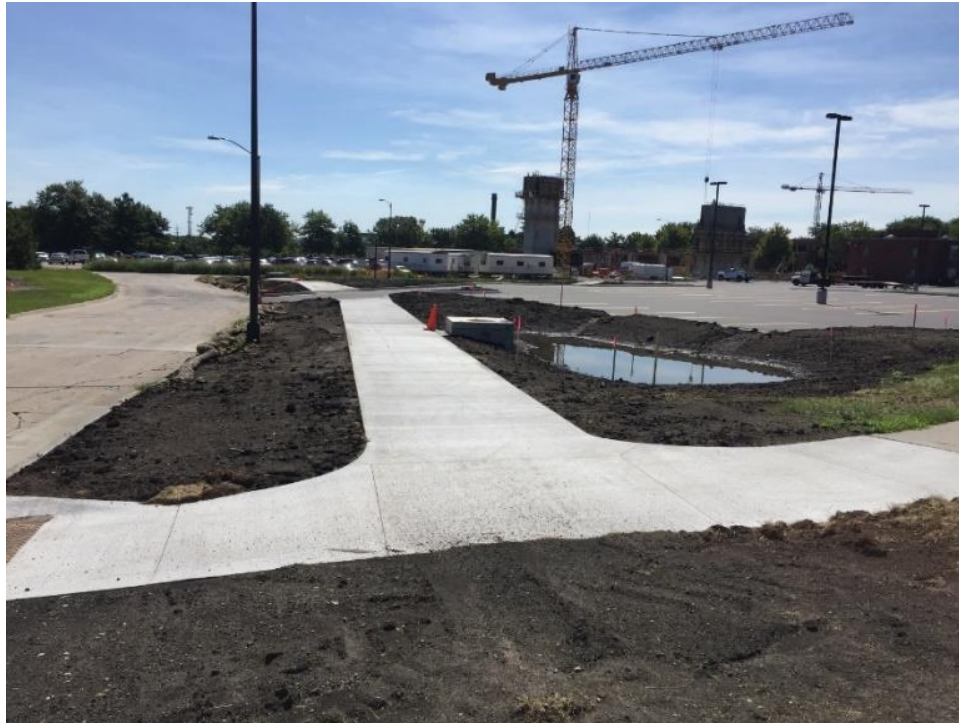
Figure 5. Constructed sidewalk (IC section)
