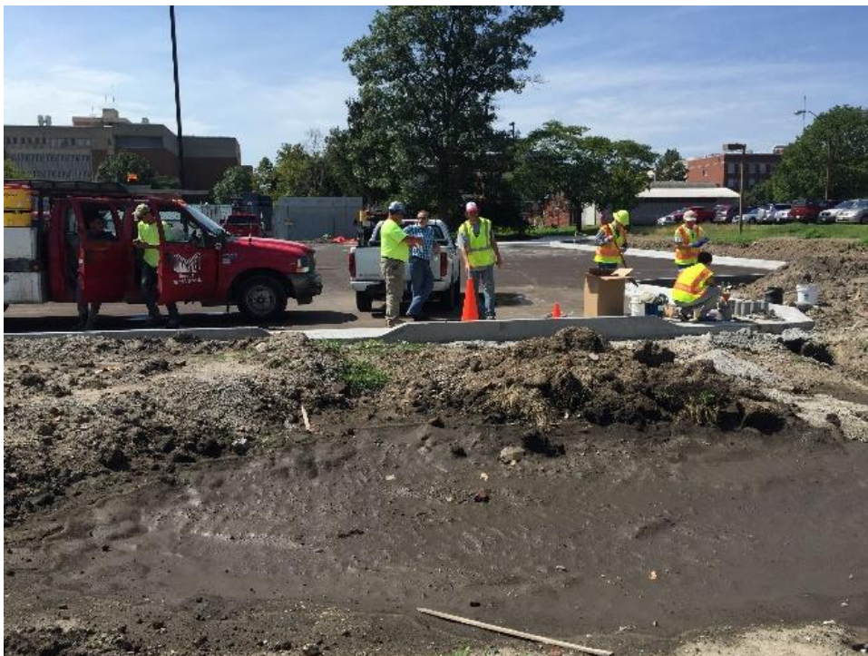
Figure 4. Obtaining test specimens in the field
