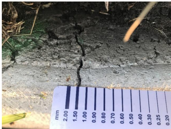
Figure 53. Joint 4 in the control section
