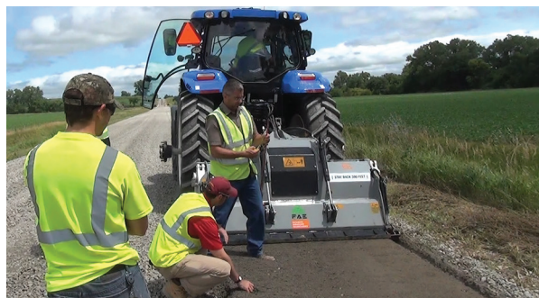
Mixing the optimized surface course materials using a reclaimer
