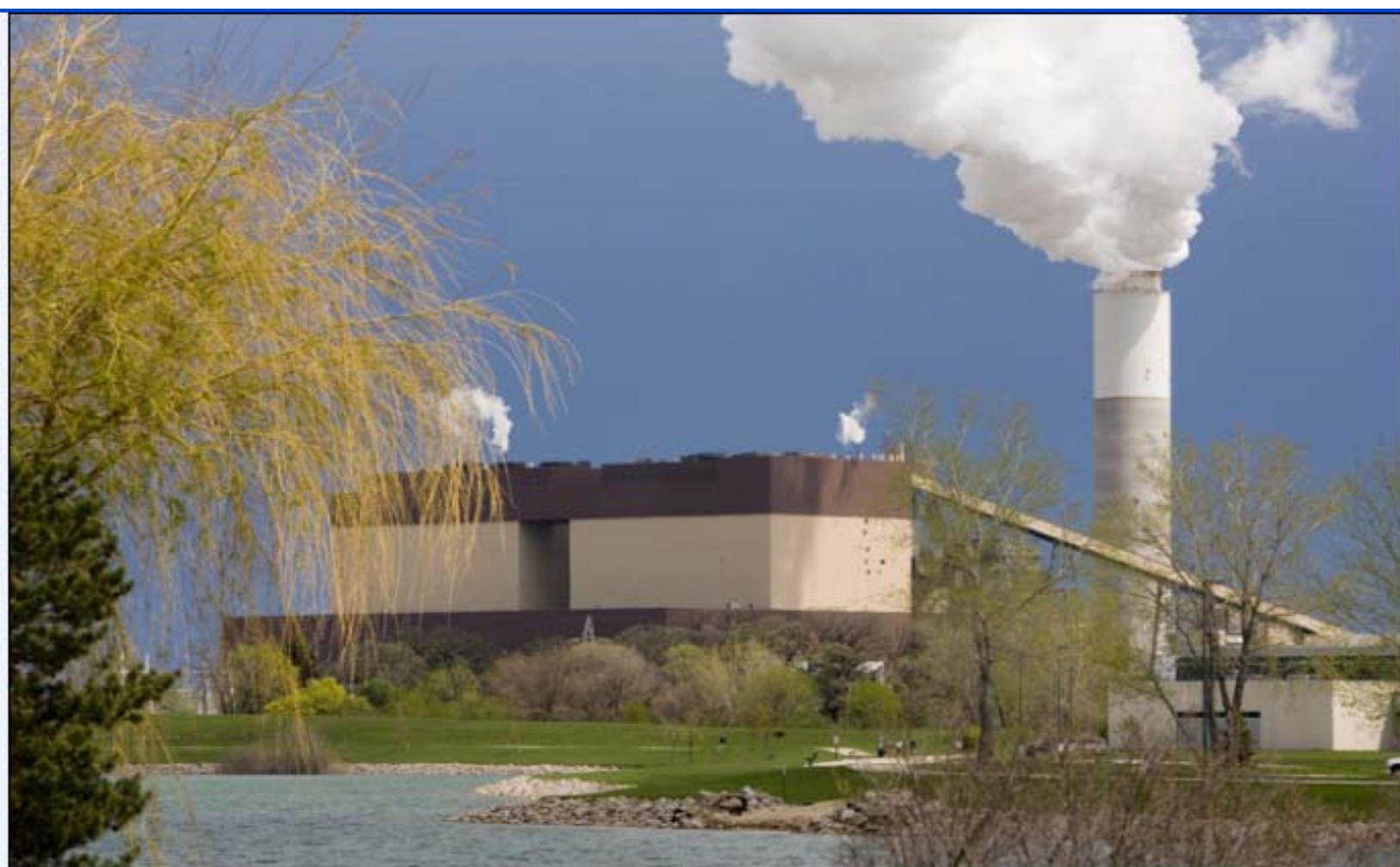
Pleasant Prairie Power Plant
