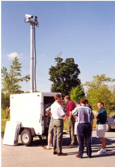
Figure 3.1. Trailer with boom partially collapsed
