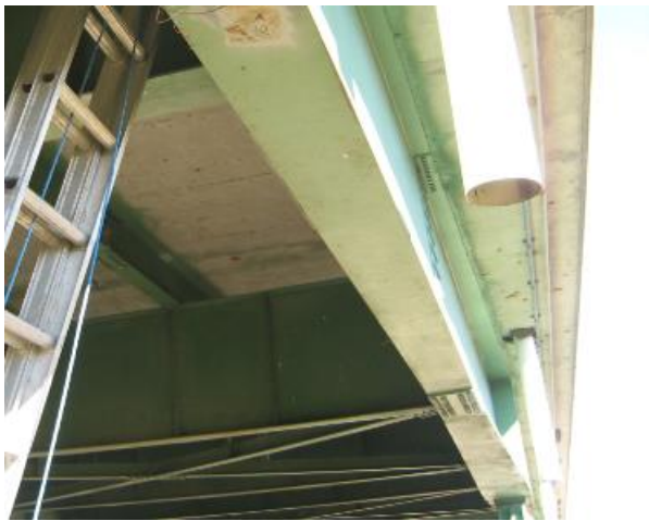
(c) South girder
