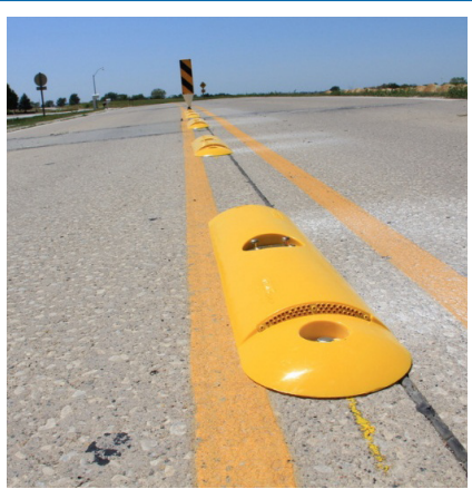
Close-up of mountable curbing
