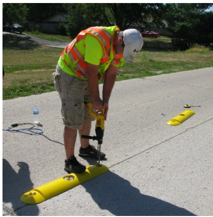
Installation of raised curbing using bolts
