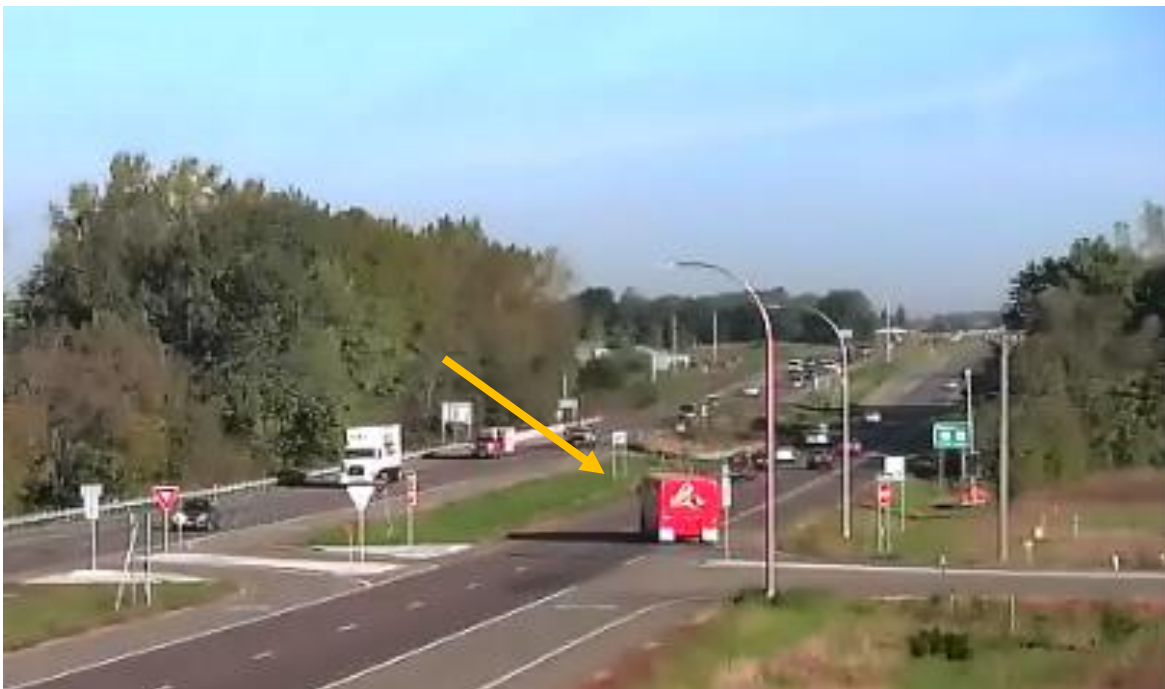
Figure 13: Truck exposure during merge from minor approach
