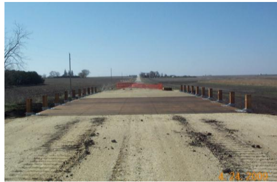
e. Plywood and guardrail posts installed
