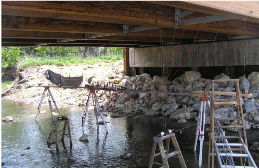
Figure 4.1. Typical instrumentation setup
