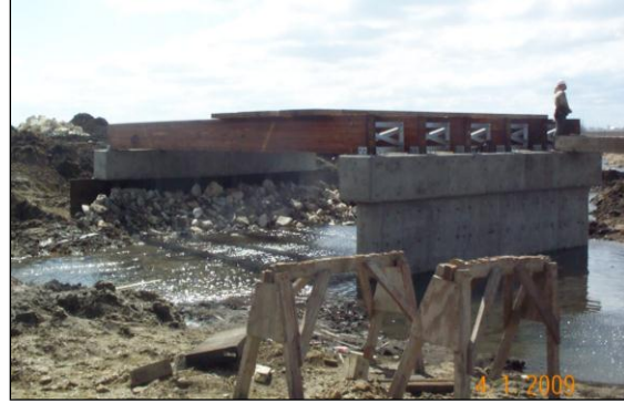
b. Erection of south span girders
