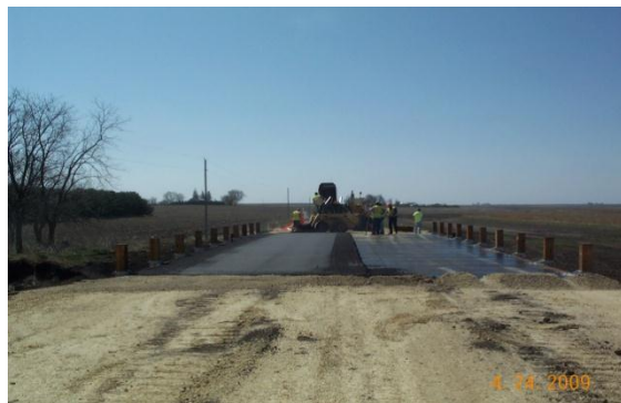
g. Placement of asphalt wearing course
