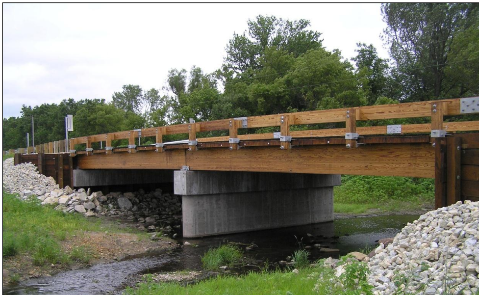
Figure 3.1. Completed demonstration bridge in service
