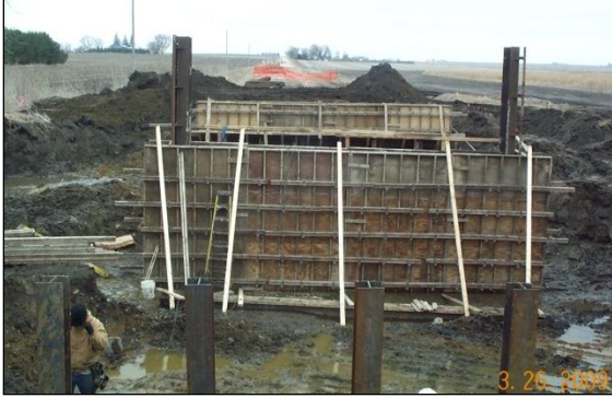
a. Construction of abutments and pier
