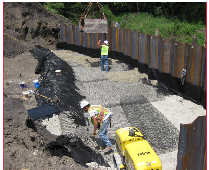
Geogrid material for Boone County west abutment
