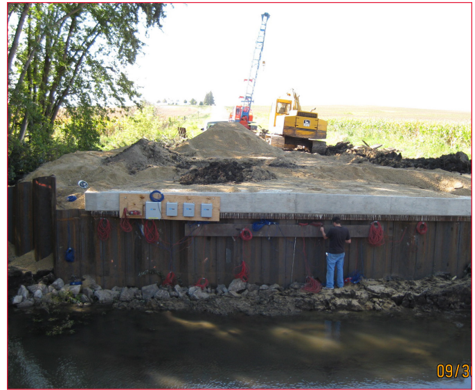
Sheet pile abutment and foundation cap with instrumentation placement
