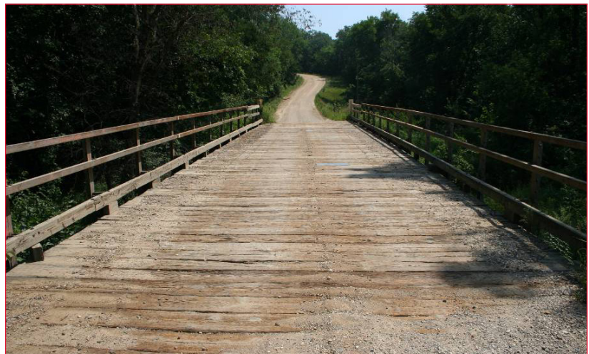
Bridge replaced for Boone County demonstration
