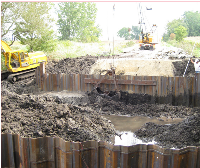
Cofferdam placement and alignment
