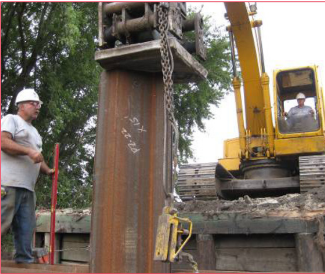
Driving of sheet pile sections with vibratory plate-equipped excavator boom
