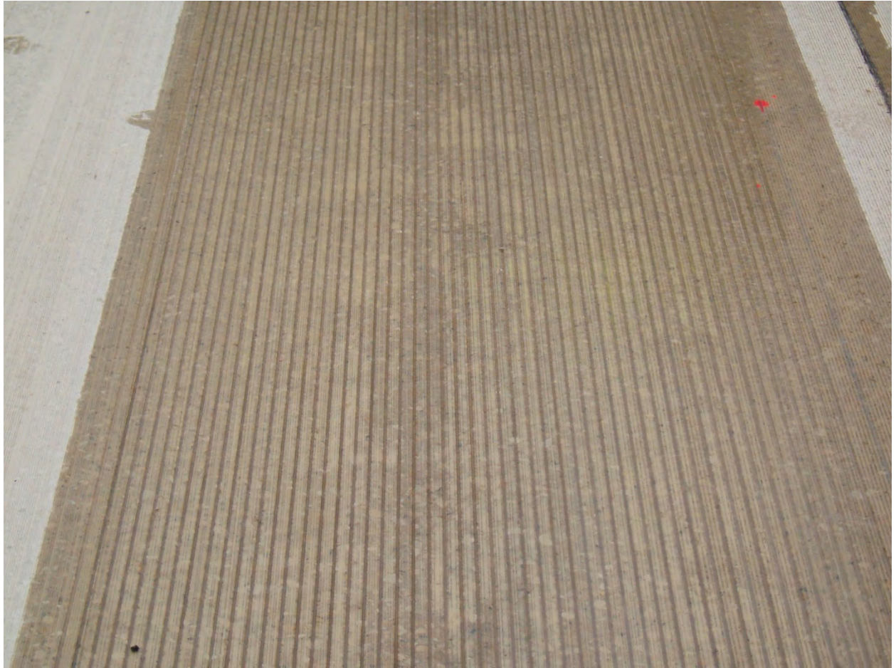
Figure 16. Next Generation surface (3/4" c-c; 1/4" deep)
