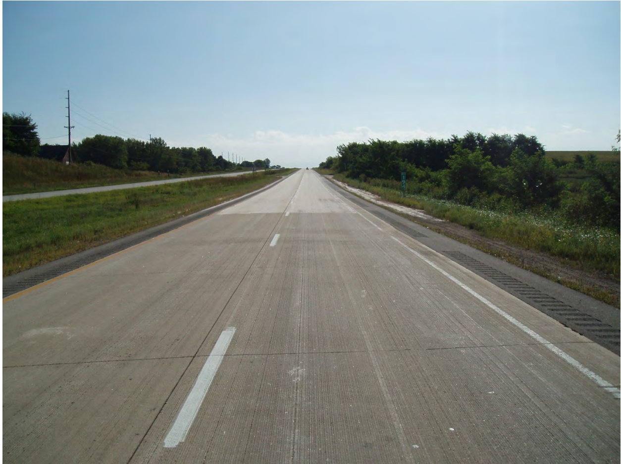
Figure 17. View of existing texture, Next Generation, grind and groove and grind only surfaces (milepost 149)
