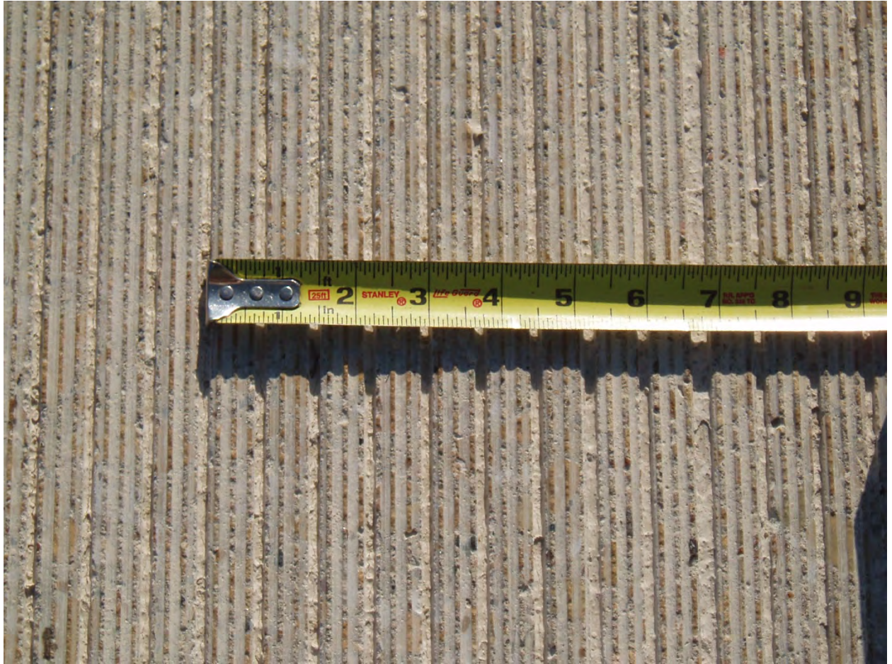
Figure 22. Ground and grooved detailed surface texture
