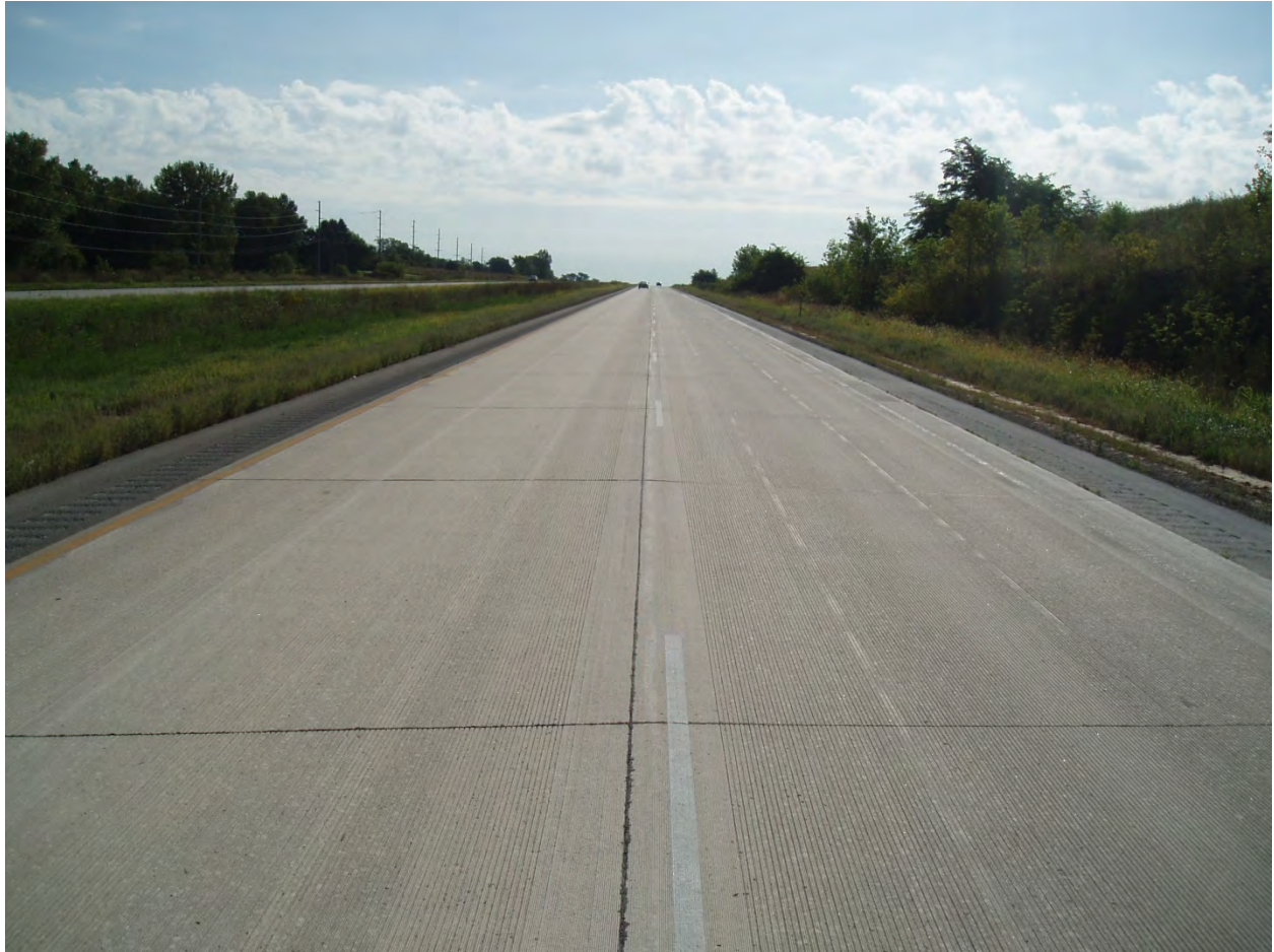
Figure 23. Ground and grooved pavement surface area
