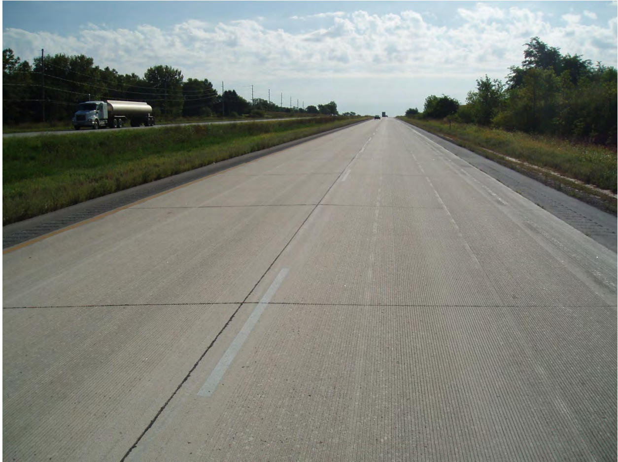
Figure 21. Ground and grooved surface test section
