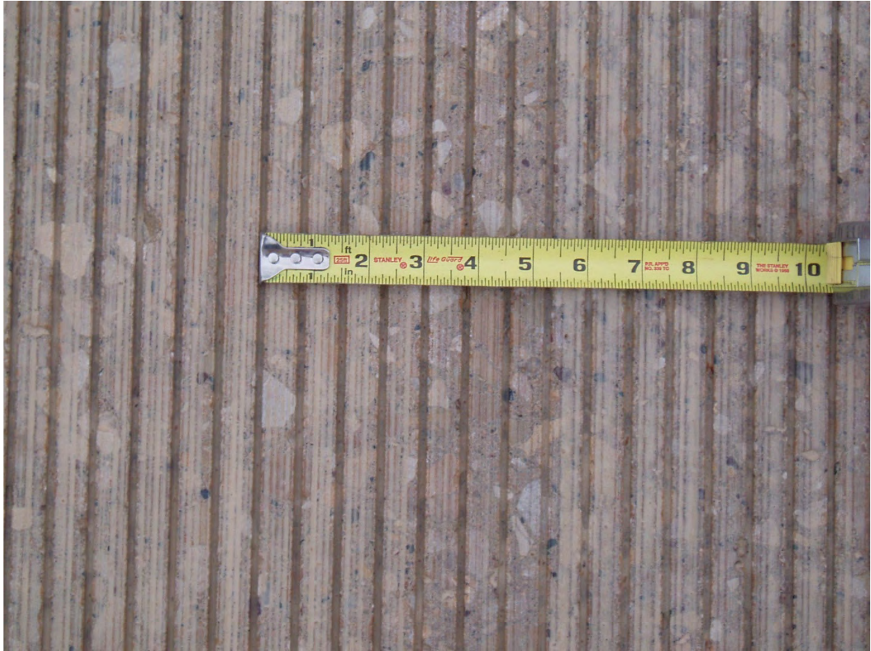
Figure 15. Next Generation grooved (3/4" c-c blades) and ground surface
