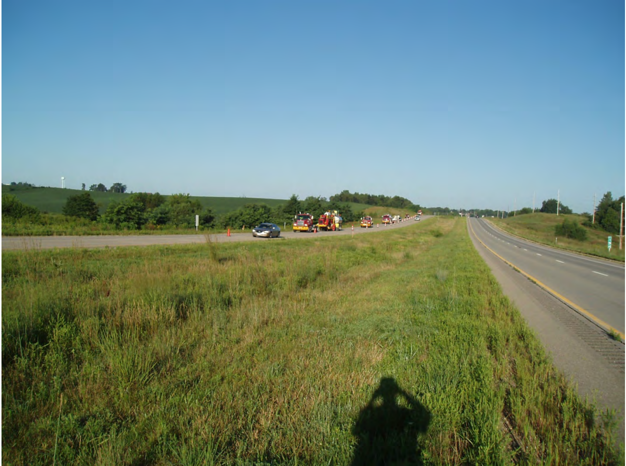
Figure 1. Surface texturing train in place on day one
