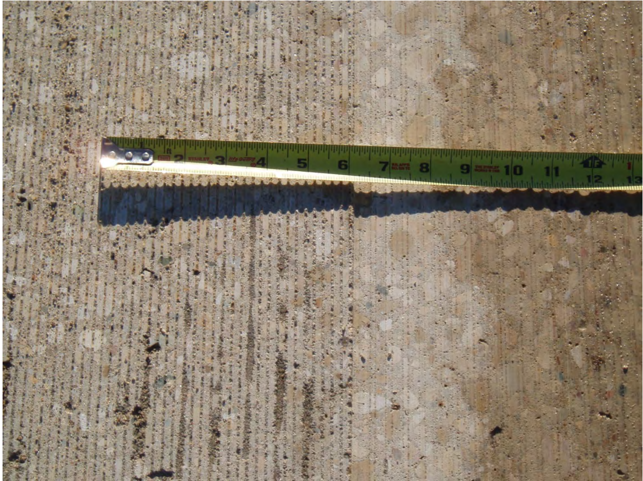
Figure 12. Standard grind vs. fine grind surface
