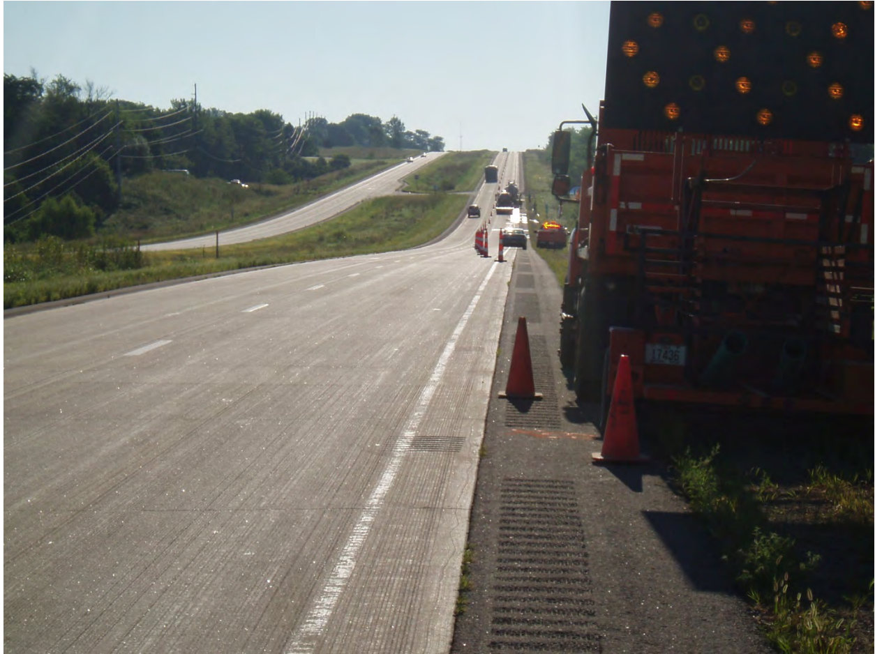
Figure 8. Typical traffic control for stage one and two construction
