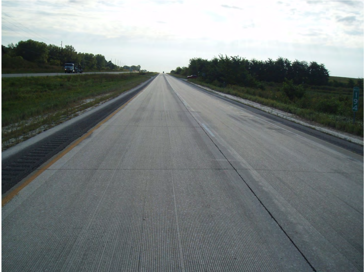
Figure 18. New Next Generation surface test section
