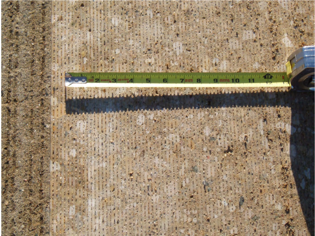
Figure 5. Standard ground surface texture
