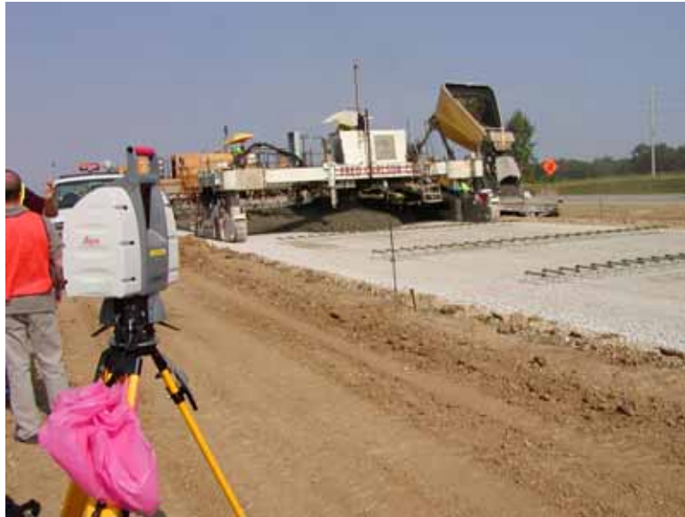
Figure 15. Performing laser scan on the subbase level
