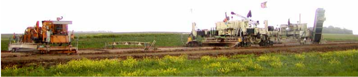
Figure 9. Paving train from Cedar Valley Corp. on IA-60 project
