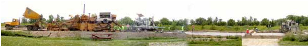
Figure 11. Paving train from Fred Carlson on G-61
