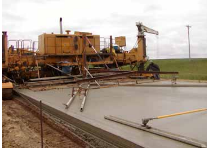
Figure 10. Jensen Co. paver with the V-float
