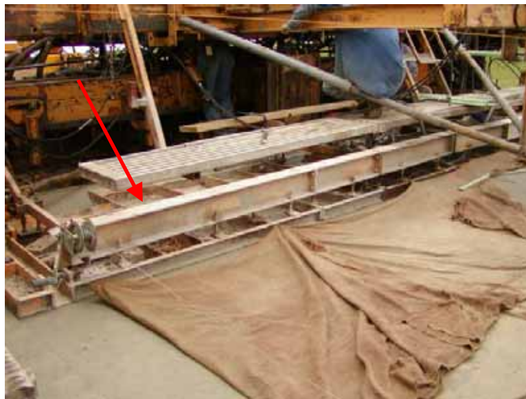
Figure 58. Possible location for ultrasonic contact sensor
